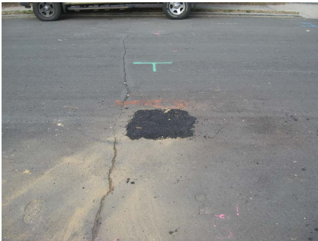
View of repaired test hole (asphalt patch).
