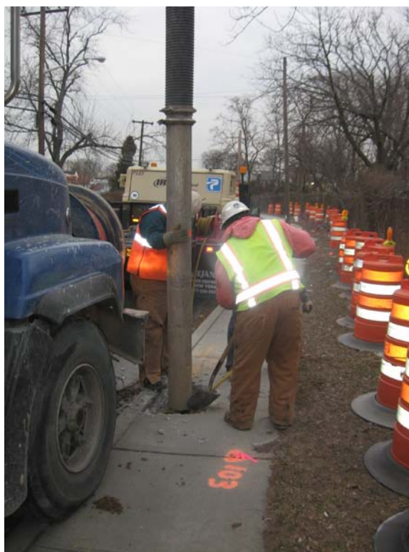
Posillico vacuuming material from test hole along Albany Ave, looking north.
