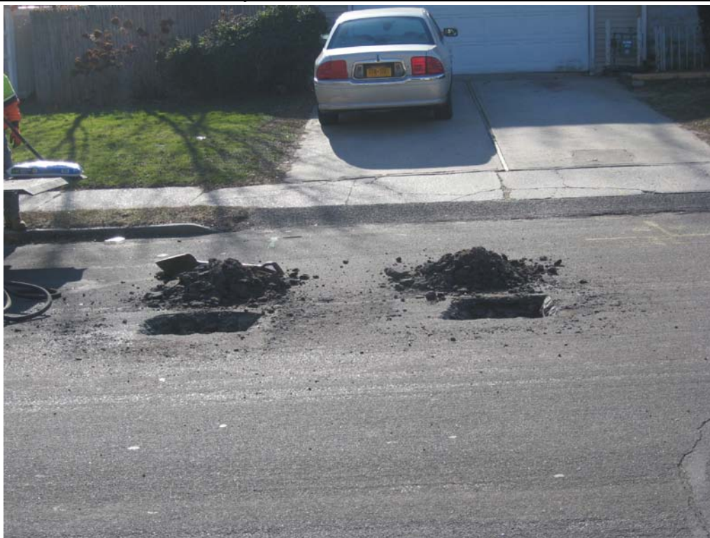
Asphalt removed from two test-hole locations via jack hammer.
