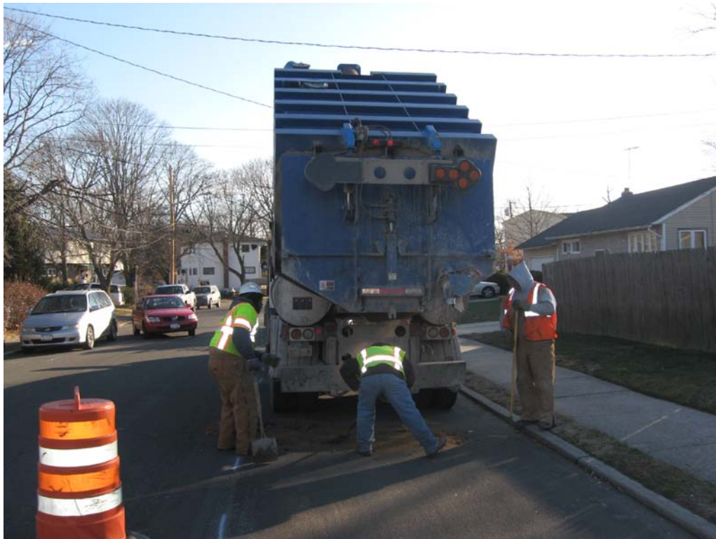
Posillico backfilling test hole via vacuum truck.
