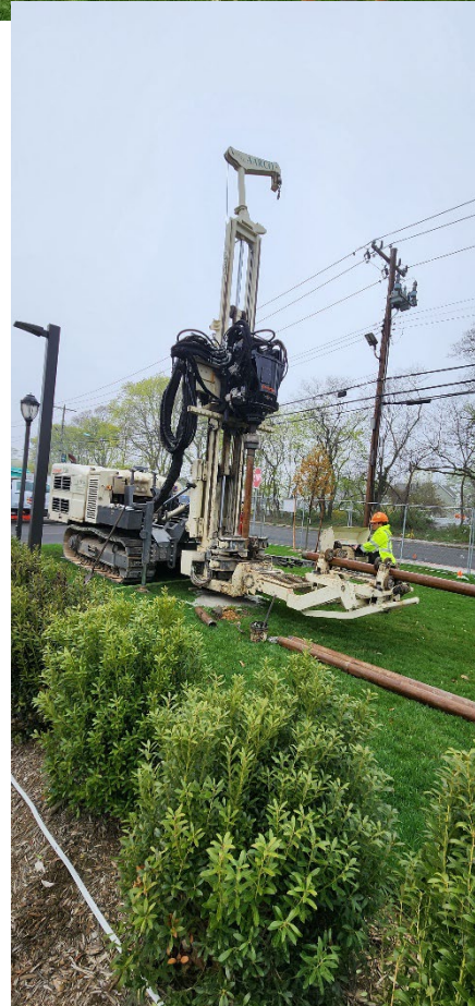
Above and Right: Setting up the sonic rig to install MW- and MW-17A on the north side of the site.
