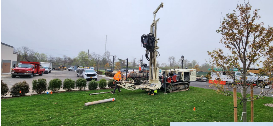
Above and Right: Setting up the sonic rig to install MW- and MW-17A on the north side of the site.
