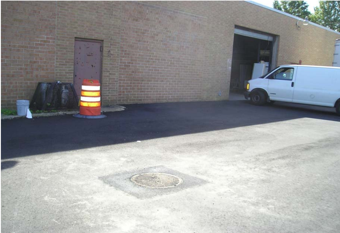
P1010001.jpg - Asphalt repaired around CP-3B, 51 Cabot St.
