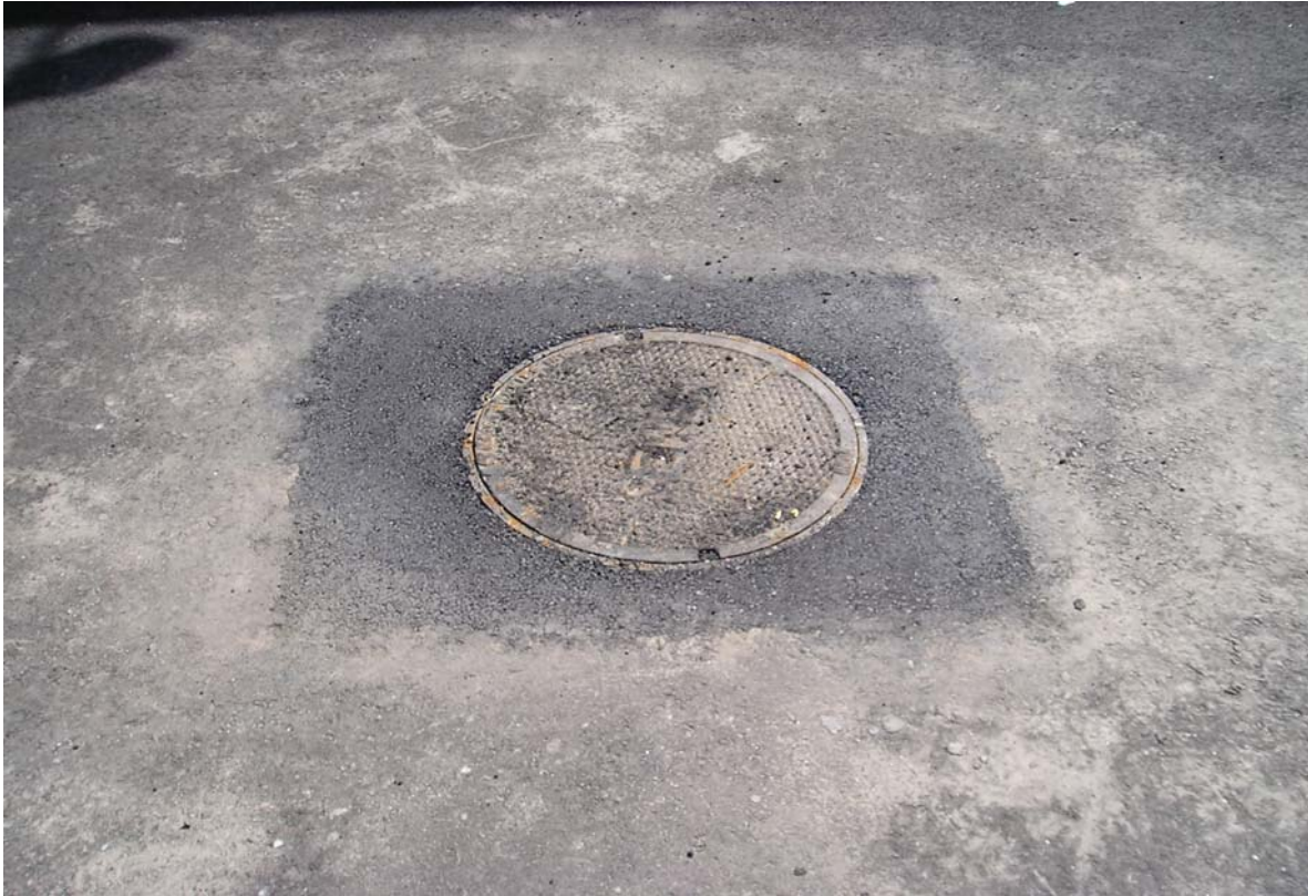
P1010002.jpg.jpg - Close up of repaired asphalt around CP-3B, 51 Cabot St.
