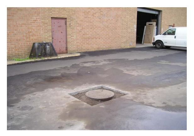
P1010007.jpg - CP-3B manhole cover at the end of the work. Permanent asphalt repair to be done.
