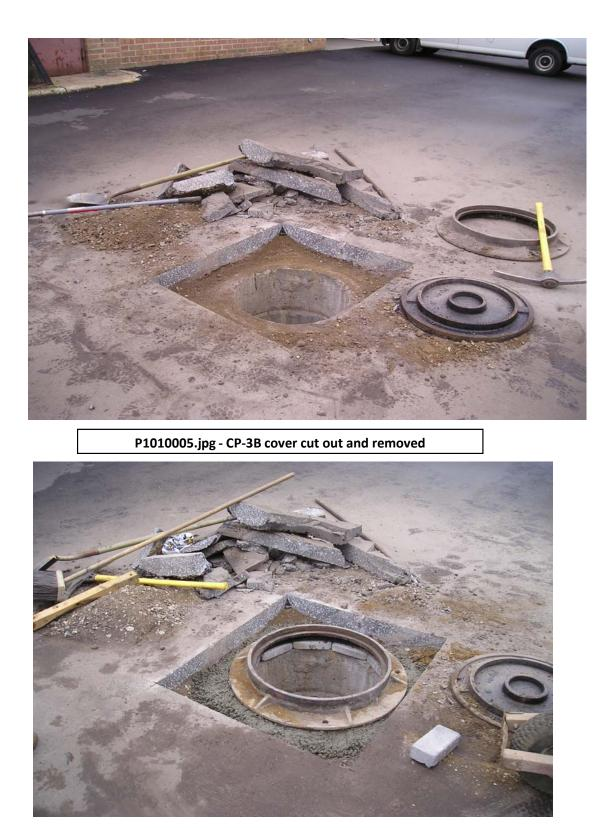
P1010006.jpg - CP-3B cover re-installed and level with existing asphalt
