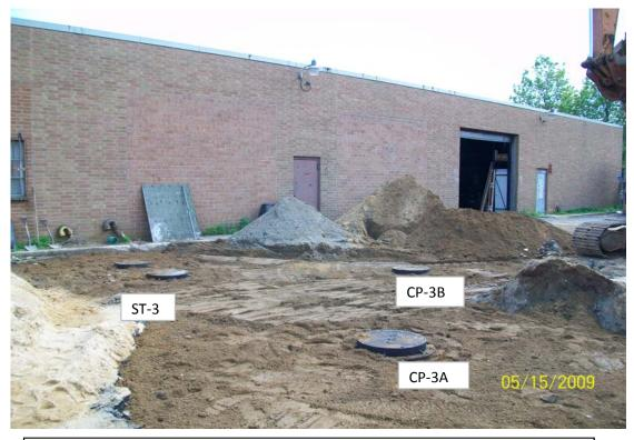
100\_0613.jpg - Completed installation of septic system #3, 51 Cabot St.
