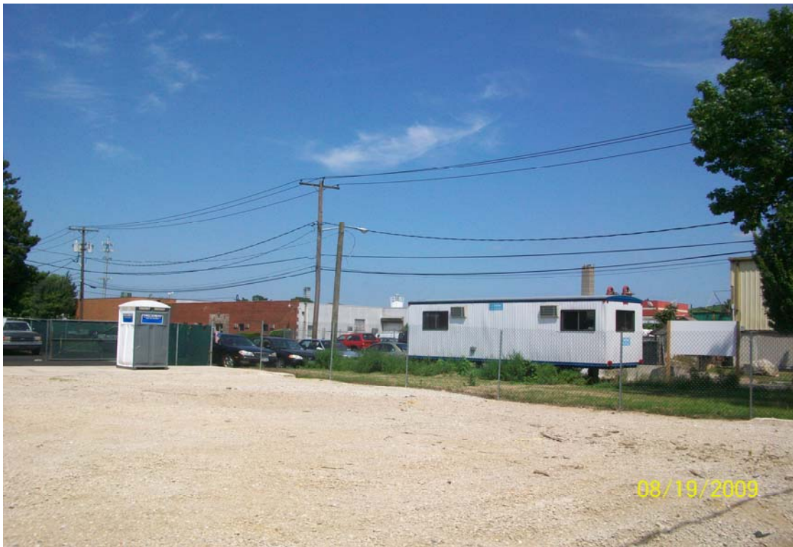
100_1193.jpg - Field trailer and port-a-john still on-site.
