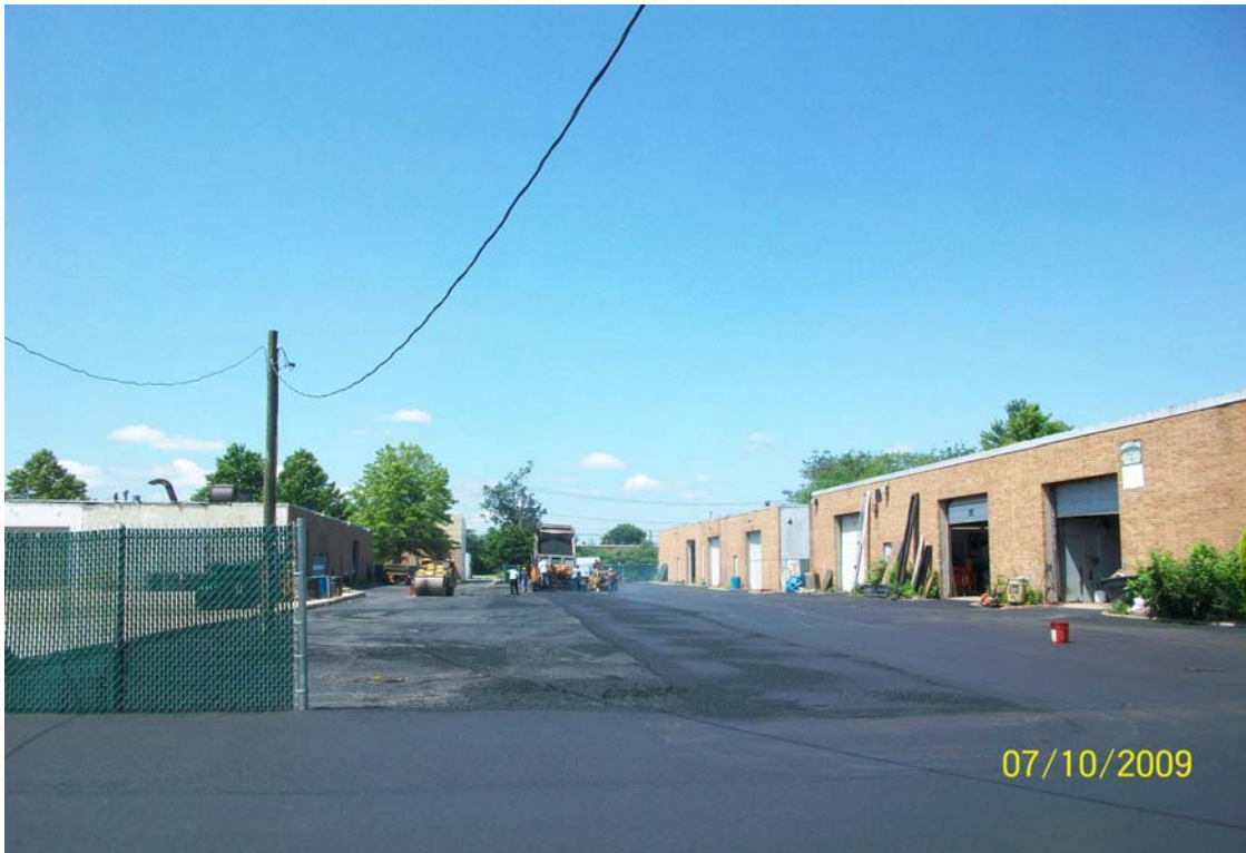
100_0949.jpg - Accurate paving from Dale St. towards Cabot St.
