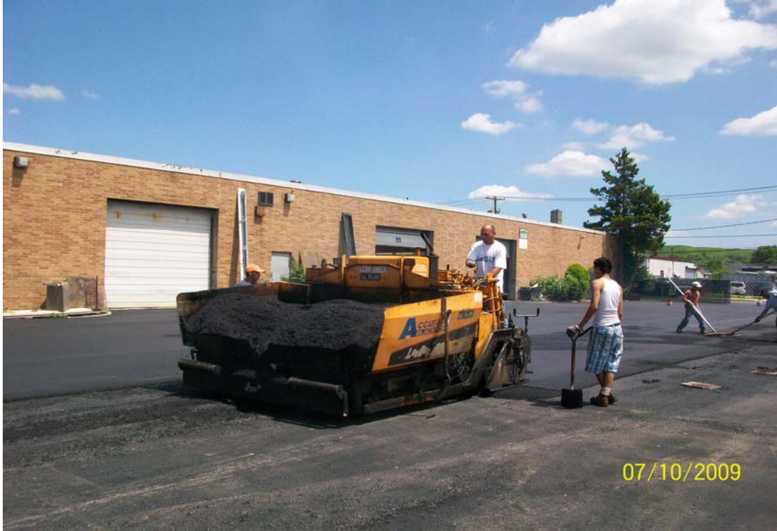
100_0950.jpg - Accurate paving from Dale St. towards Cabot St.
