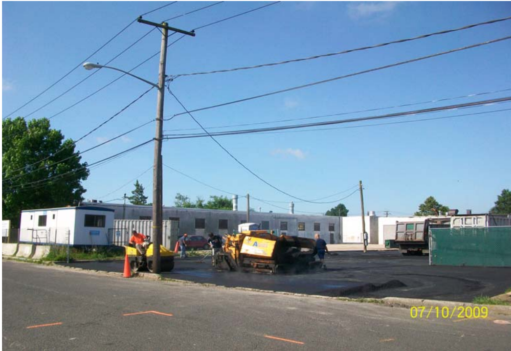
100_0948.jpg - Accurate Blacktop starting to pave 1.5" wear course by Dale St.
