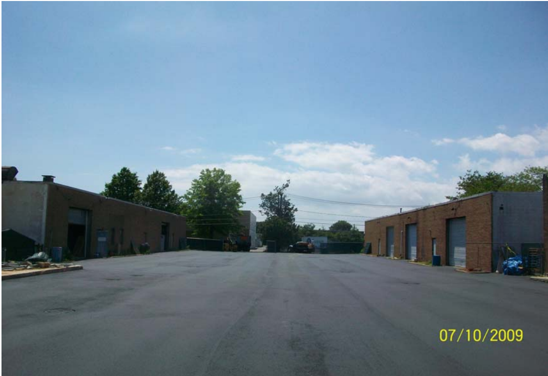
100_0951.jpg - Accurate finished paving the 51/61 Cabot St. are, looking west
