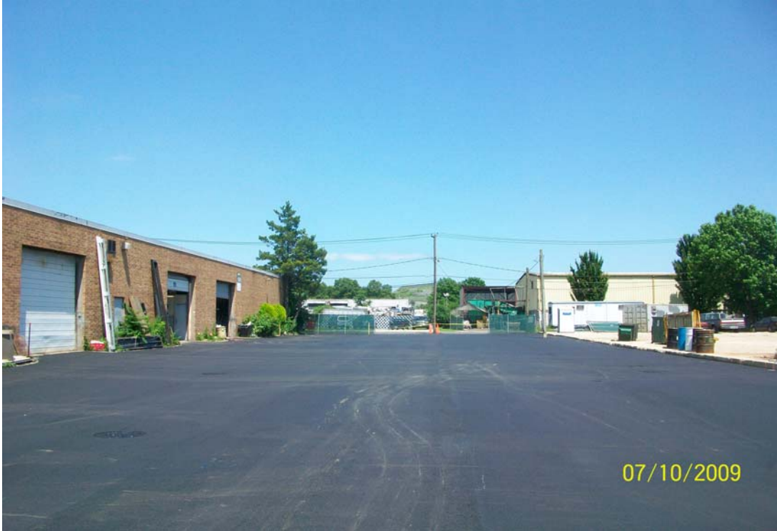
100_0951.jpg - Accurate finished paving the 50/60 Dale St. area, looking east
