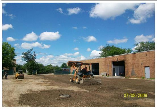
100\_0940.jpg - Accurate Blacktop spreading RCA at 61 Cabot St.
