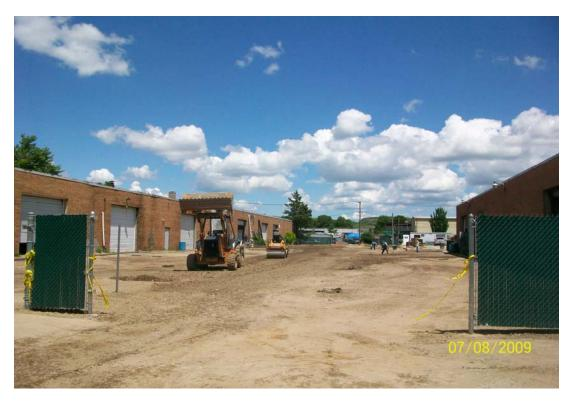
100\_0941 - Accurate Blacktop grading and compacting RCA, looking east
