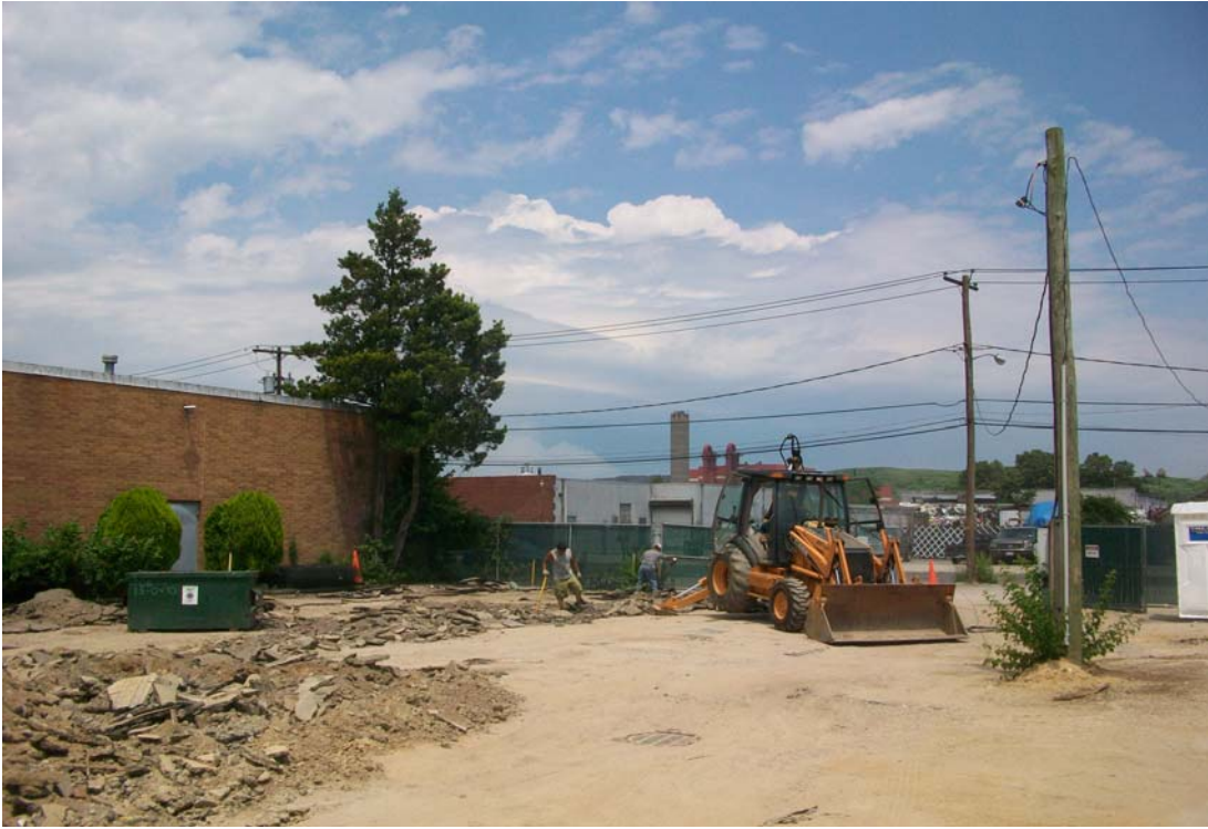
100_0928.jpg - Accurate Blacktop removing asphalt from 60 Dale St.
