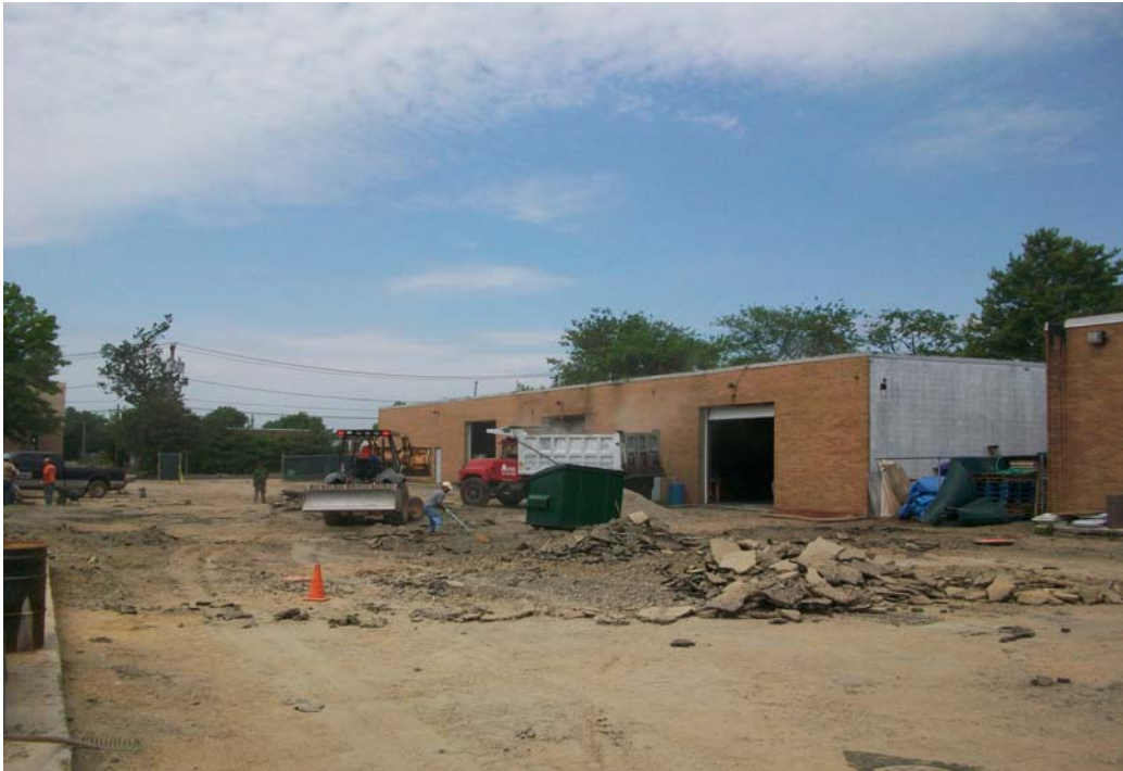
100_0926.jpg - Accurate Blacktop removing asphalt Cabot and Dale St. areas
