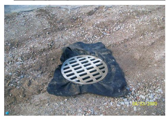
100 0854.jpg - New filter fabric installed on new drainage structure cover
