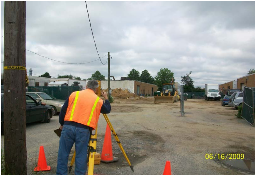
100-0833.jpg - YEC surveyors surveying the UST-5/9 excavation
