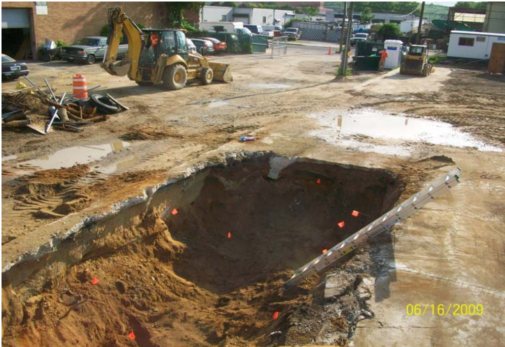
100_0829.jpg - UST-5/9 excavation with sample locations
