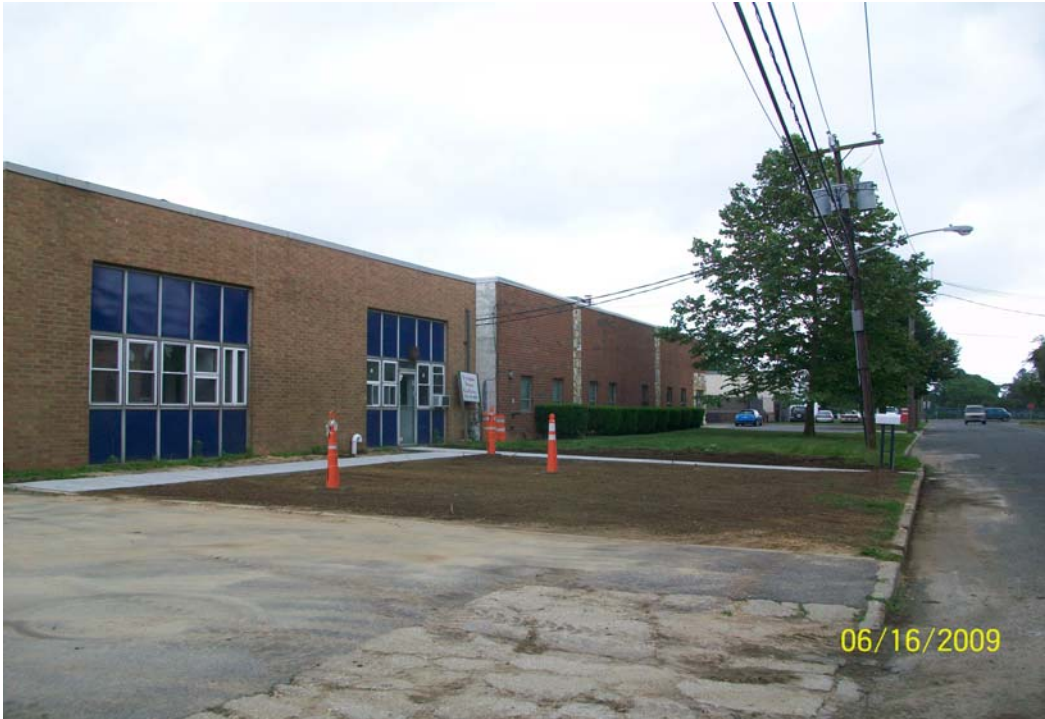
100_0835.jpg - Finished cleaning and grading before topsoil/seeding 61 Cabot St.
