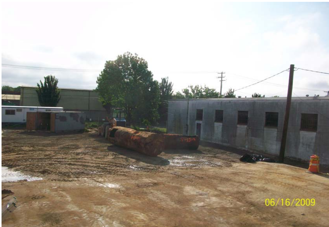
100_0830.jpg - Removed UST-5 and 9 tanks awaiting disposal, looking east
