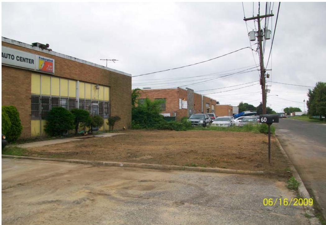
100_0834.jpg - Finished cleaning and grading before topsoil/seeding 60 Dale St.
