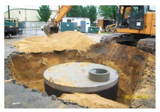
100\_0785.jpg - PDS-9, 60 Dale St., being backfilled
