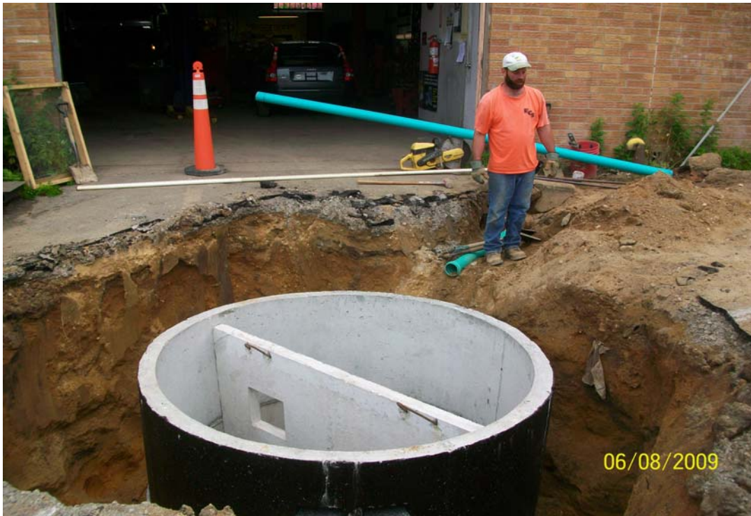
100_0775.jpg - PST-5, 60 Dale St., tank and baffle wall installed
