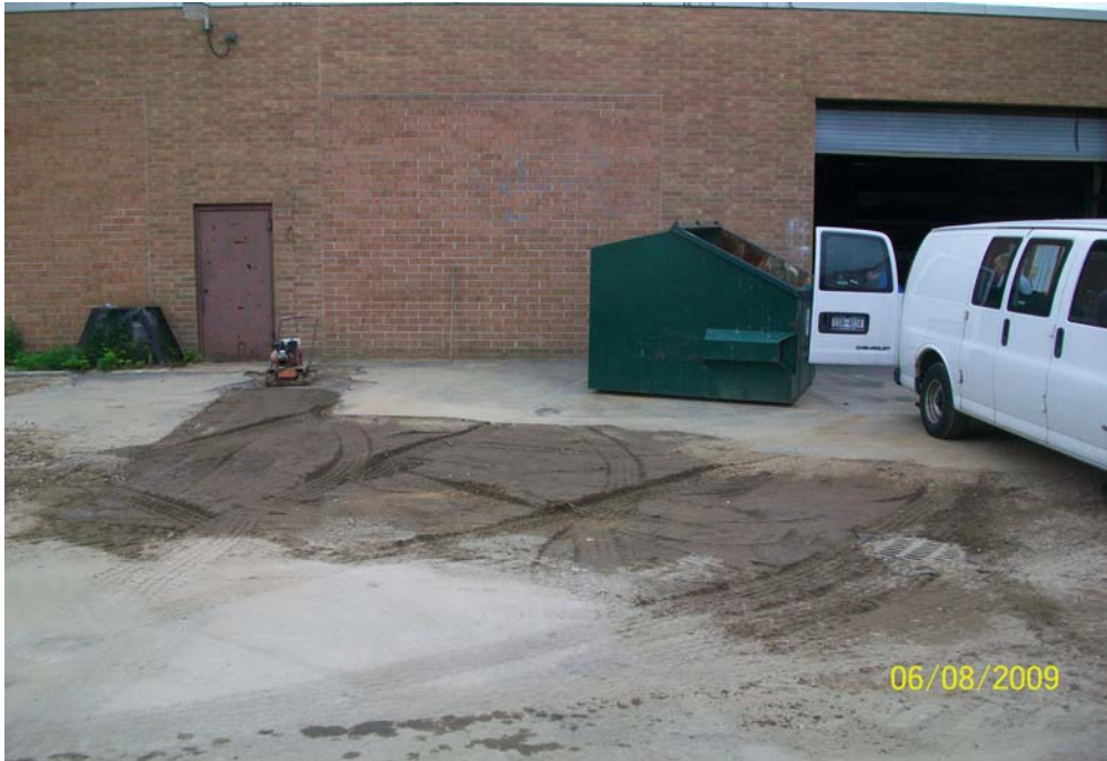
100_0771.jpg - DS-5, 51 Cabot St., abandonment completed
