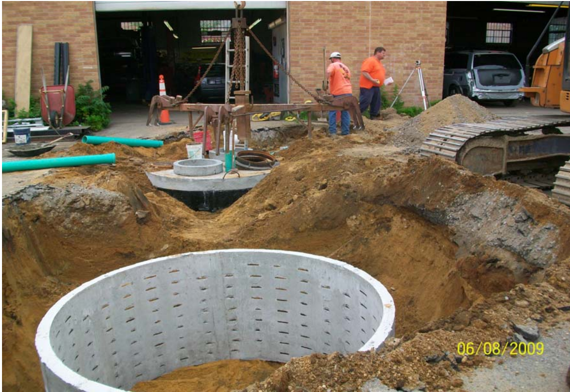
100_0778.jpg - PCP-5A, 60 Dale St., structure installed
