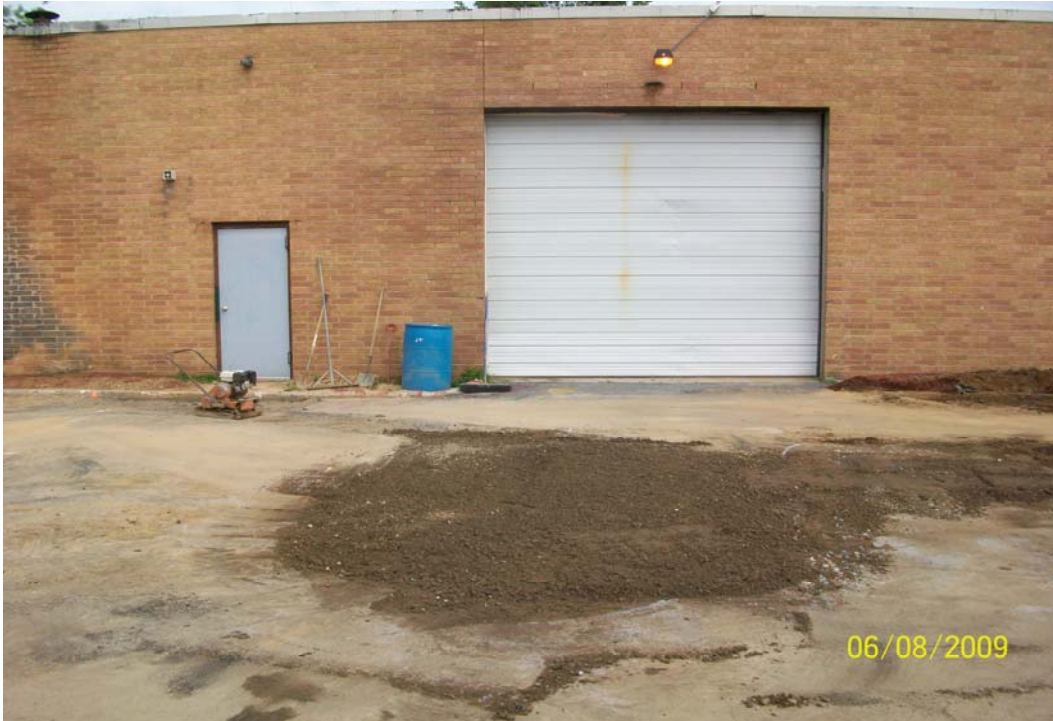
100_0774.jpg - DS-4, 61 Cabot St., abandonment completed
