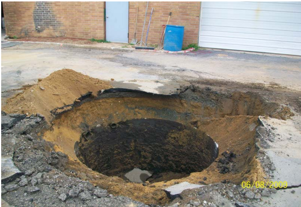
100_0773.jpg - DS-4, 61 Cabot St., partially abandoned
