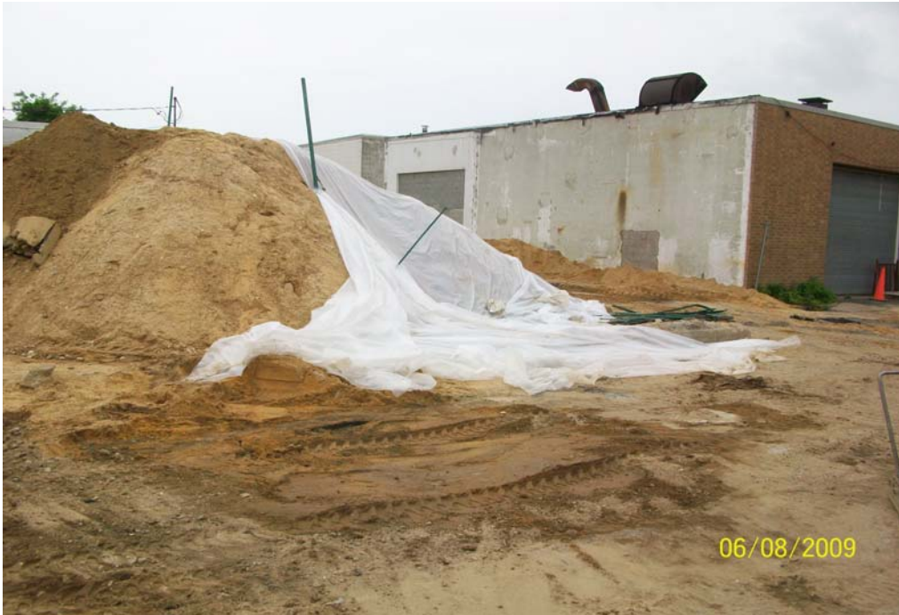
100_0777.jpg - DS-8, 50 Dale St., abandonment completed
