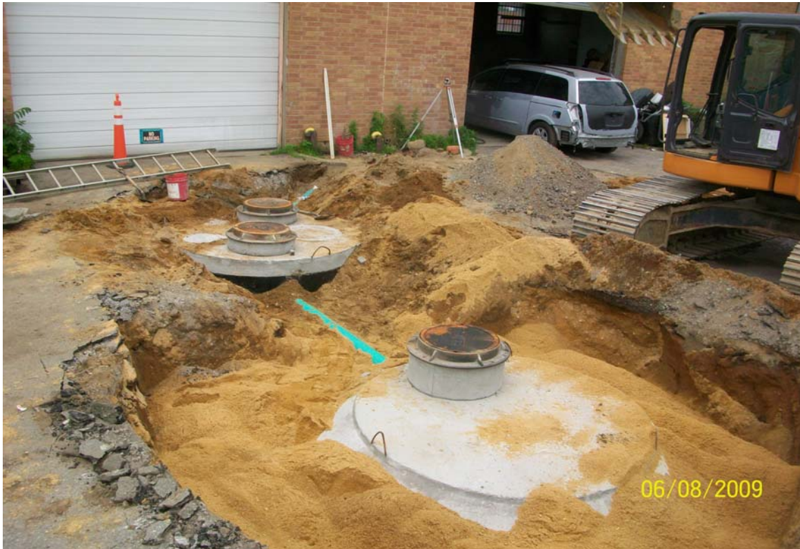
100_0779.jpg - PST-5, PCP-5A and piping installed, 60 Dale St.
