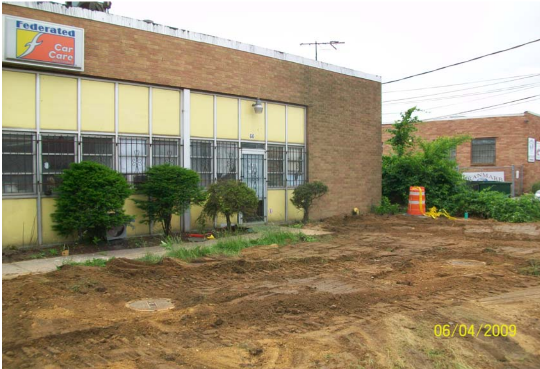
100_0759.jpg -Septic system #6, 60 Dale St., backfilled
