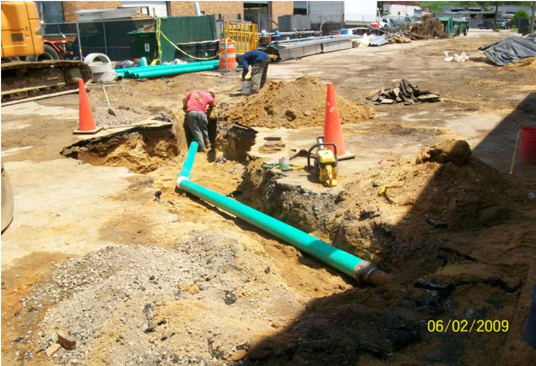
006.jpg - Roof drain #4, 51 Cabot St., connected to PDS-6
