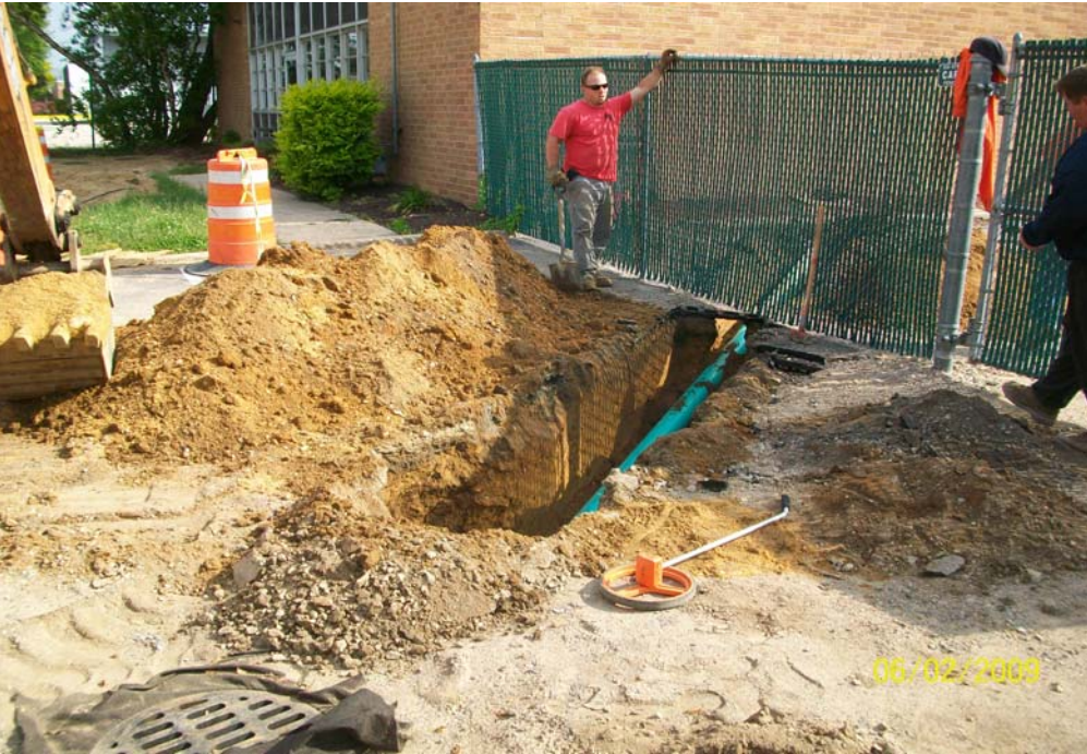
003.jpg - Roof drain #1, 61 Cabot St., connected to PDS-3 in foreground
