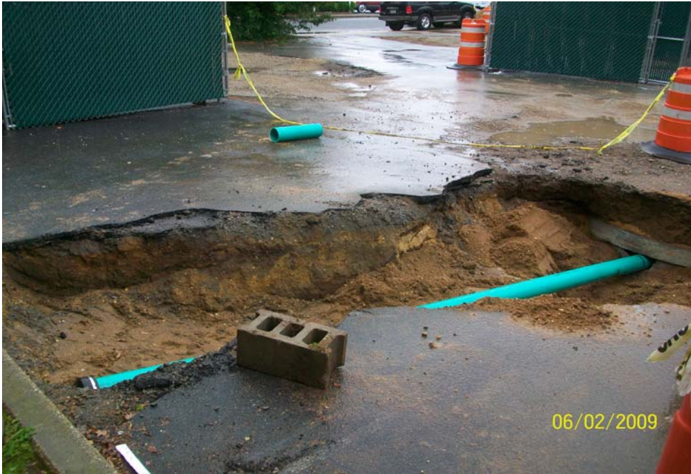
005.jpg - Roof drain #1, 51 Cabot St., connected to PDS-4
