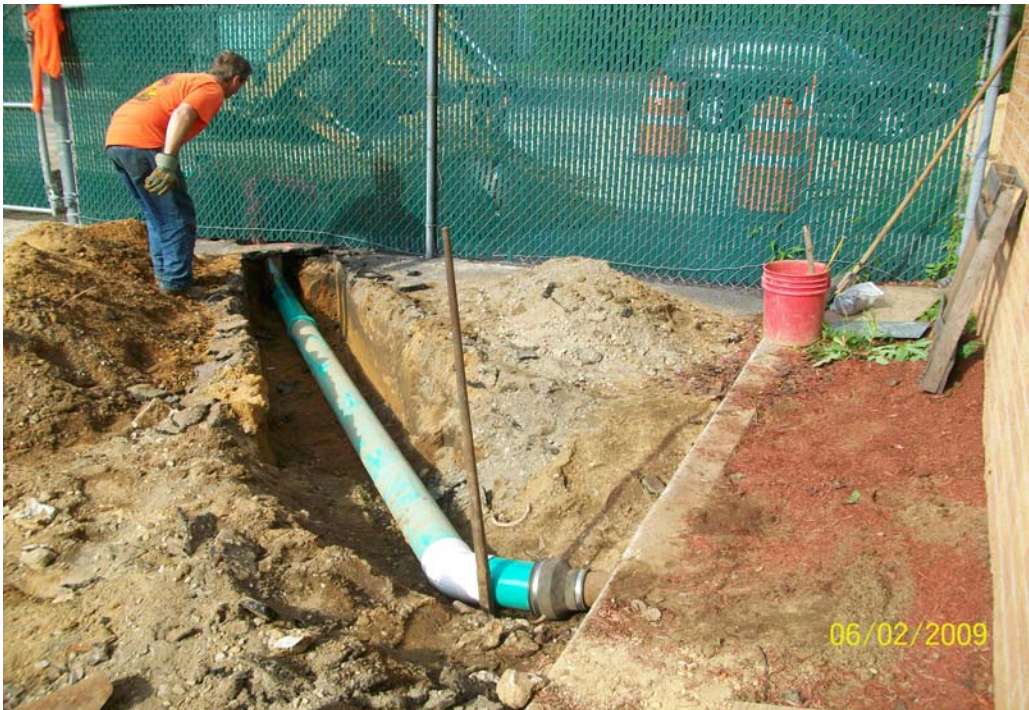
002.jpg - Roof drain #1, 61 Cabot St., connected to PDS-3
