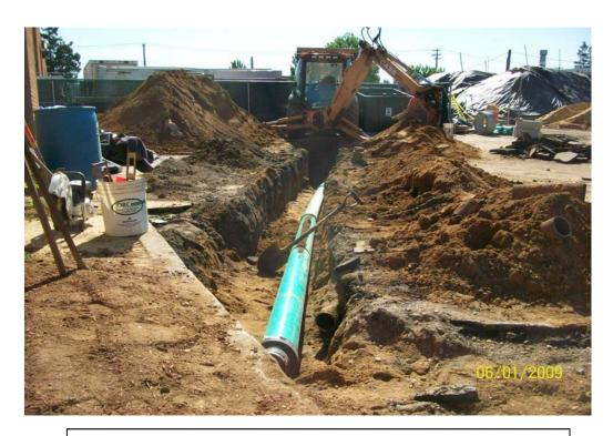
004.jpg - Cork and Sons installing roof drain #3 to PDS-3, 61 Cabot St.
