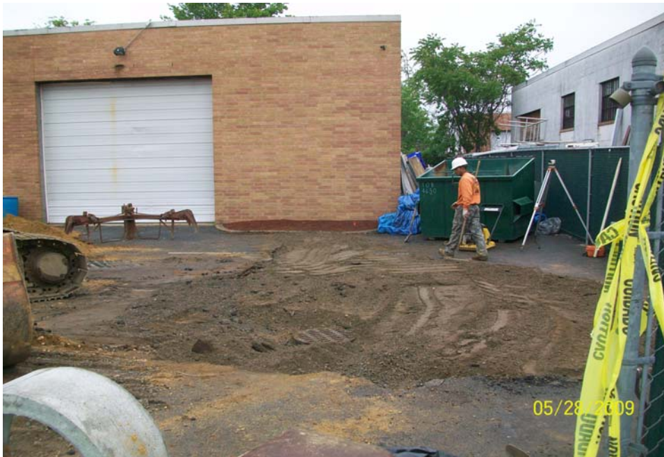
100_0724.jpg - PDS-3 and redirected roof drain backfilled
