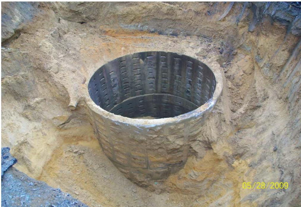
100_0712.jpg - CP-11, 61 Cabot St., partially excavated out
