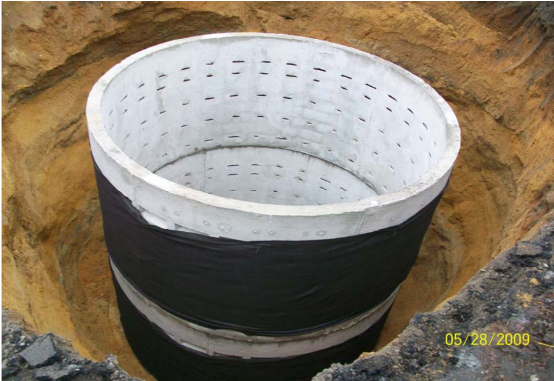
100_0717pg - PDS-3, 61 Cabot St., both rings installed
