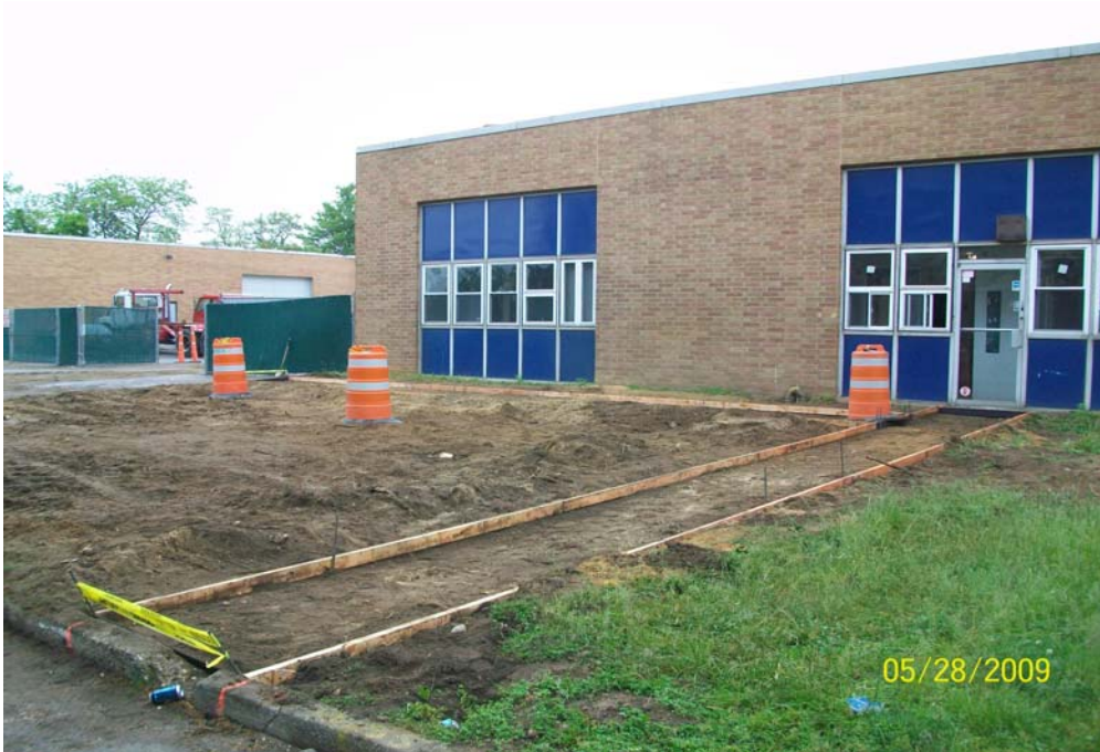
100_0721.jpg - Replacement sidewalk in front of 51 Cabot St. prepped for concrete
