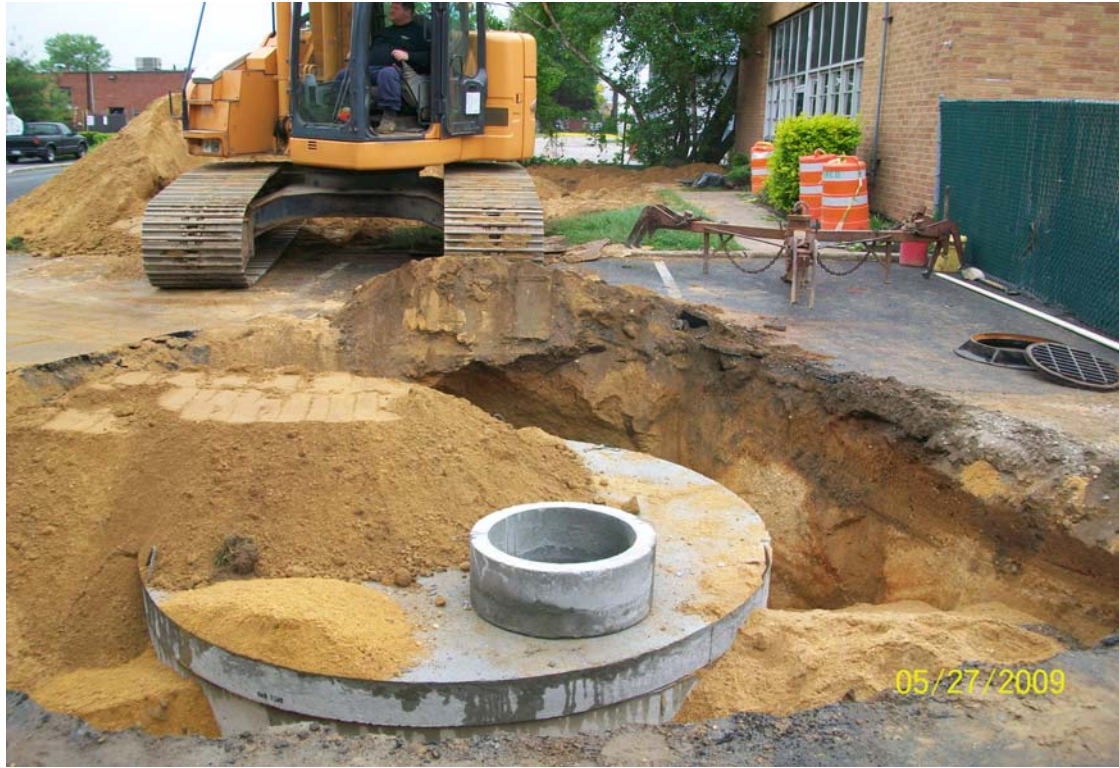
100_0685.jpg - PDS-1 partially backfilled, 61 Cabot St.
