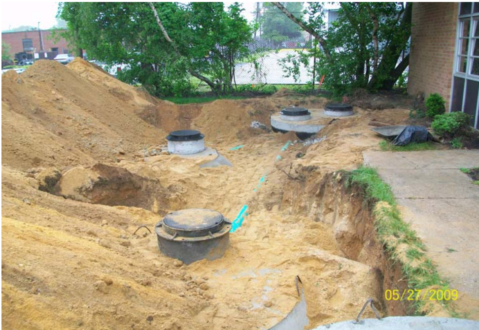
100_0703.jpg - Septic system #2 prior to backfilling, 61 Cabot St.
