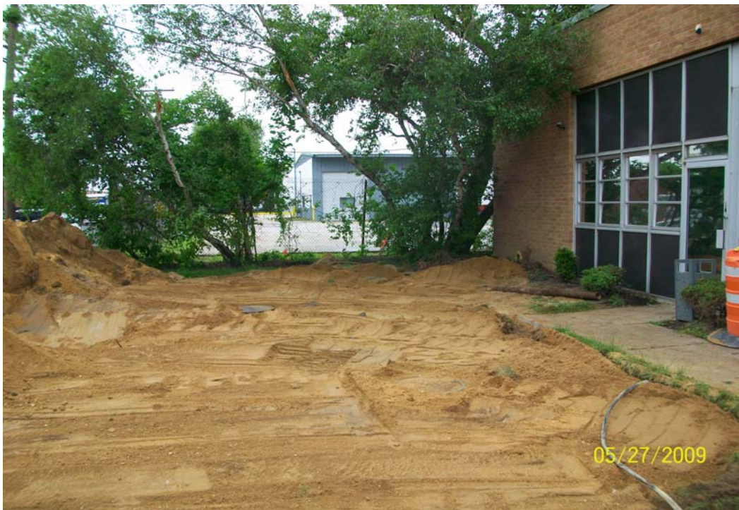
100_0705.jpg - Septic system #2 backfilled, 61 Cabot St.
