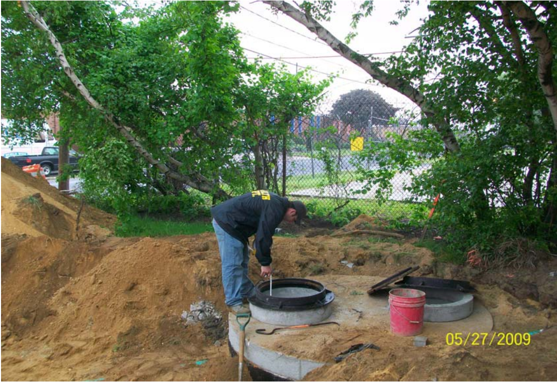
100_0701pg - Jimmy Trent (SCDHS) inspecting septic system #2, 61 Cabot St.
