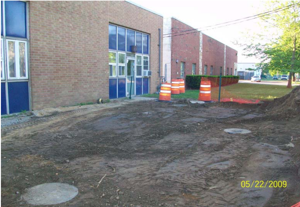
100_0666.jpg - Backfilling complete at septic system #1, 51 Cabot St.
