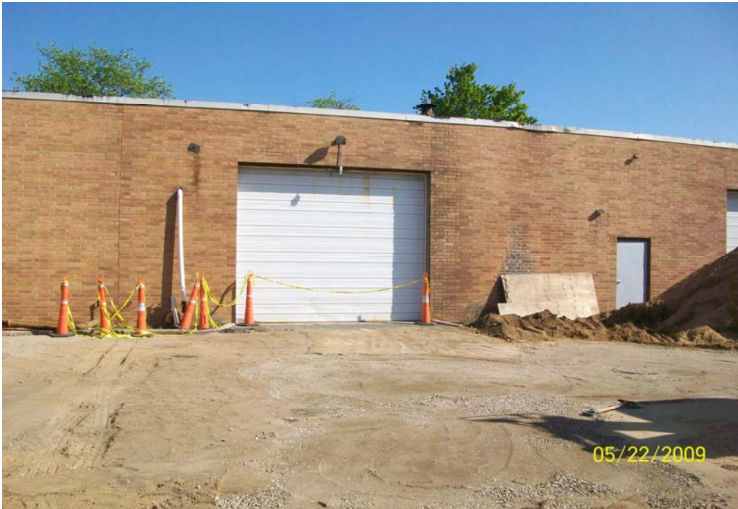
100_0667.jpg - Backfilling complete at septic system #4, 61 Cabot St.
