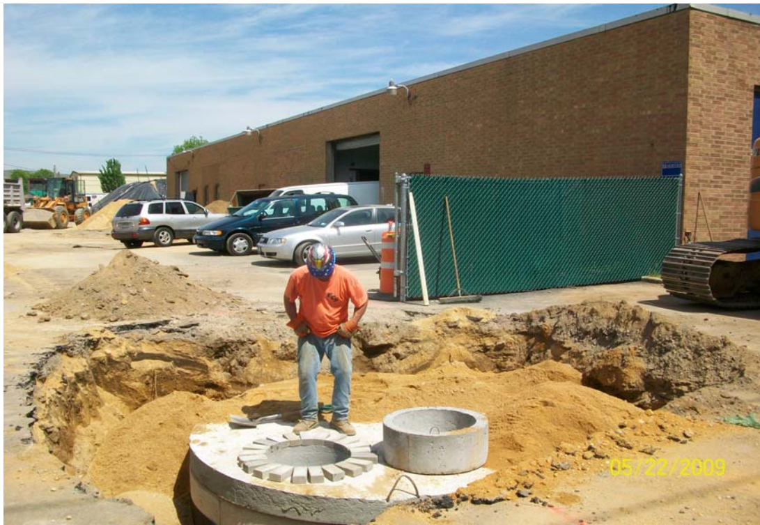
100_0676.jpg - PDS installed and partially backfilled
