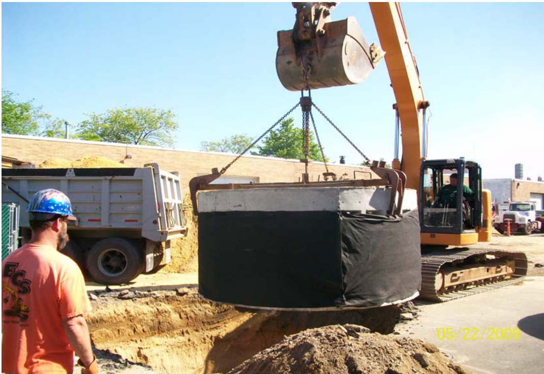
100_0668pg - Installing PDS-4 structure with filter fabric, 51 Cabot St.
