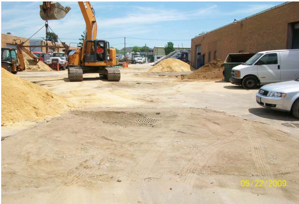
100_0670.jpg - Finished backfilling and compacting PDS-4, 51 Cabot St.
