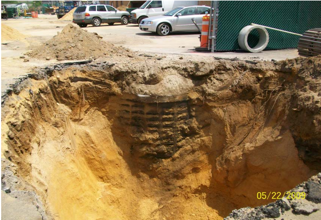
100_0675.jpg - CP-1 partially exposed, PDS-5 installed next to this
