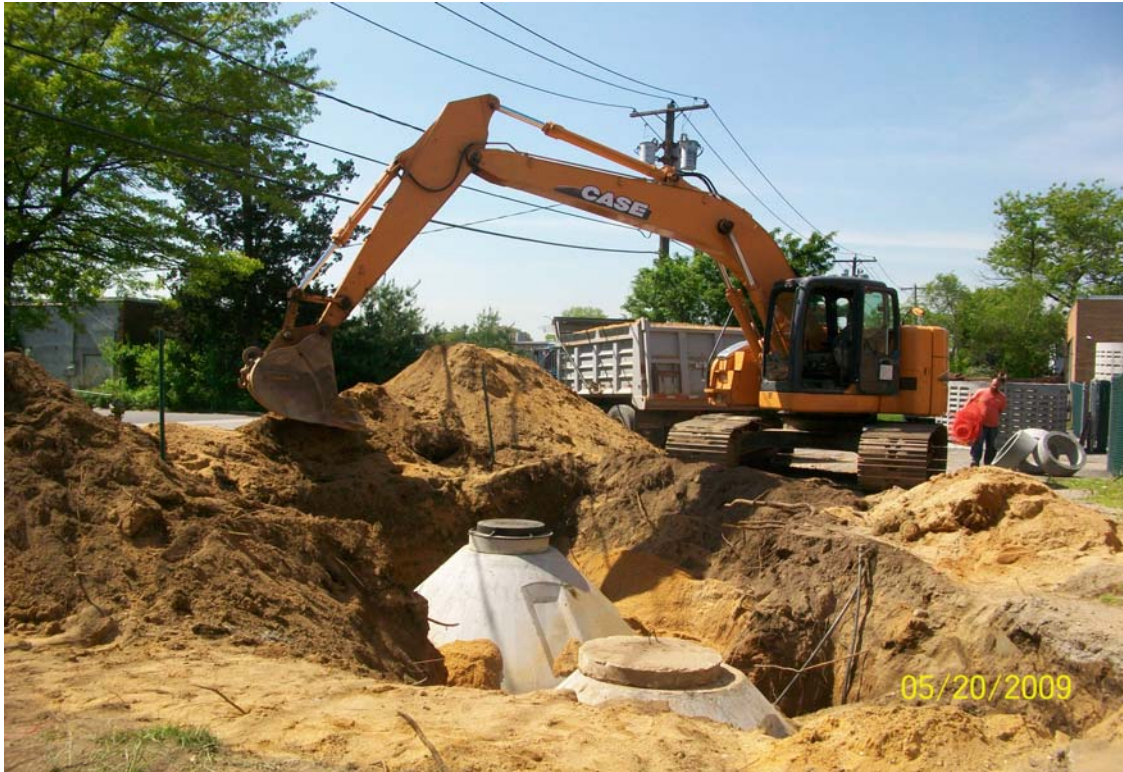
100_00648.jpg - Installation of PST-4 (foreground) and PCP-4A (background)
