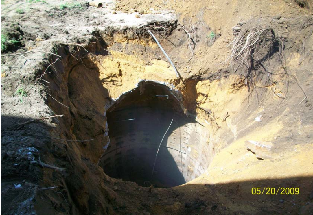
100_00640.jpg - CP-5 partially removed, in front of 51 Cabot St.
