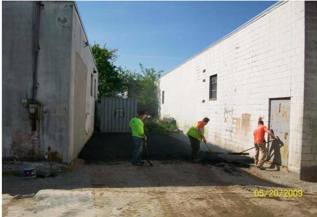
100_00639.jpg - Installing 3" binder course in south alleyway
