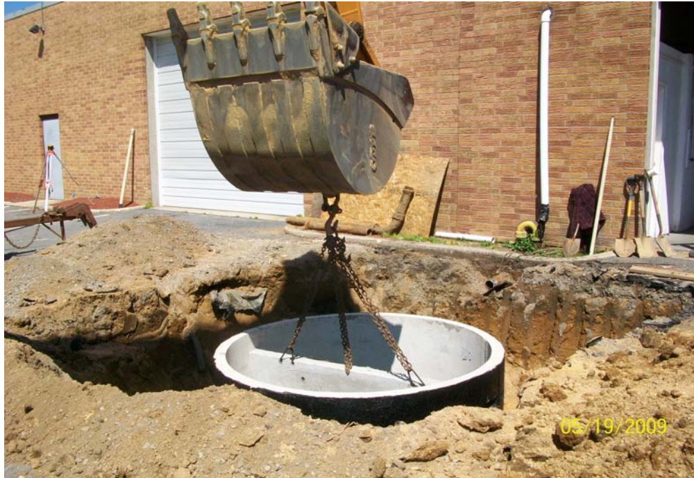
100_00632.jpg - Installing PST-1, 61 Cabot St.
