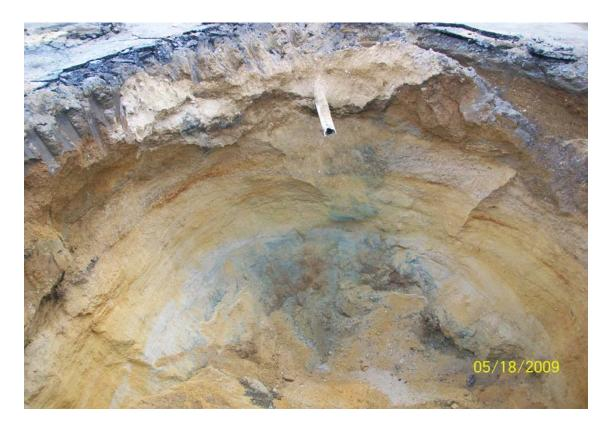
100\_00623.jpg - Visibly contaminated green soil left on south wall of CP-6A,6-12' BGS
