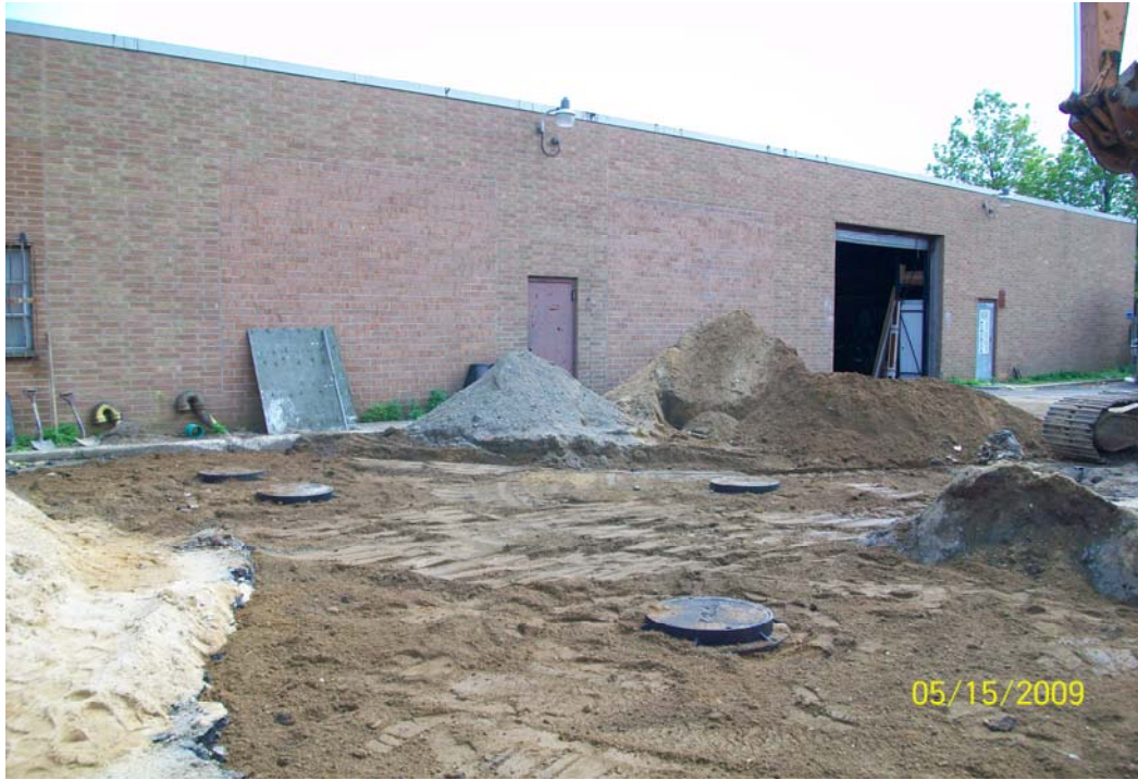
100_00614.jpg - Septic system 3 backfilled to grade
