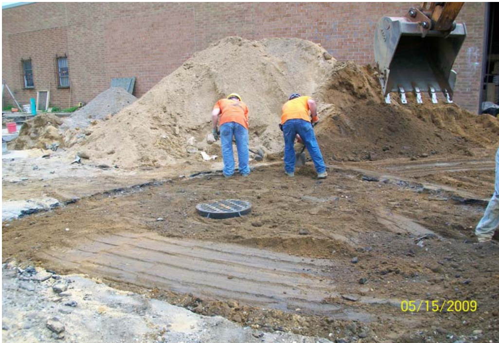
100_00613.jpg - PDS-7 backfilled to grade
