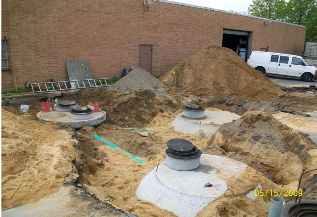
100_00612.jpg - Finished installing septic system 3 prior to inspection
