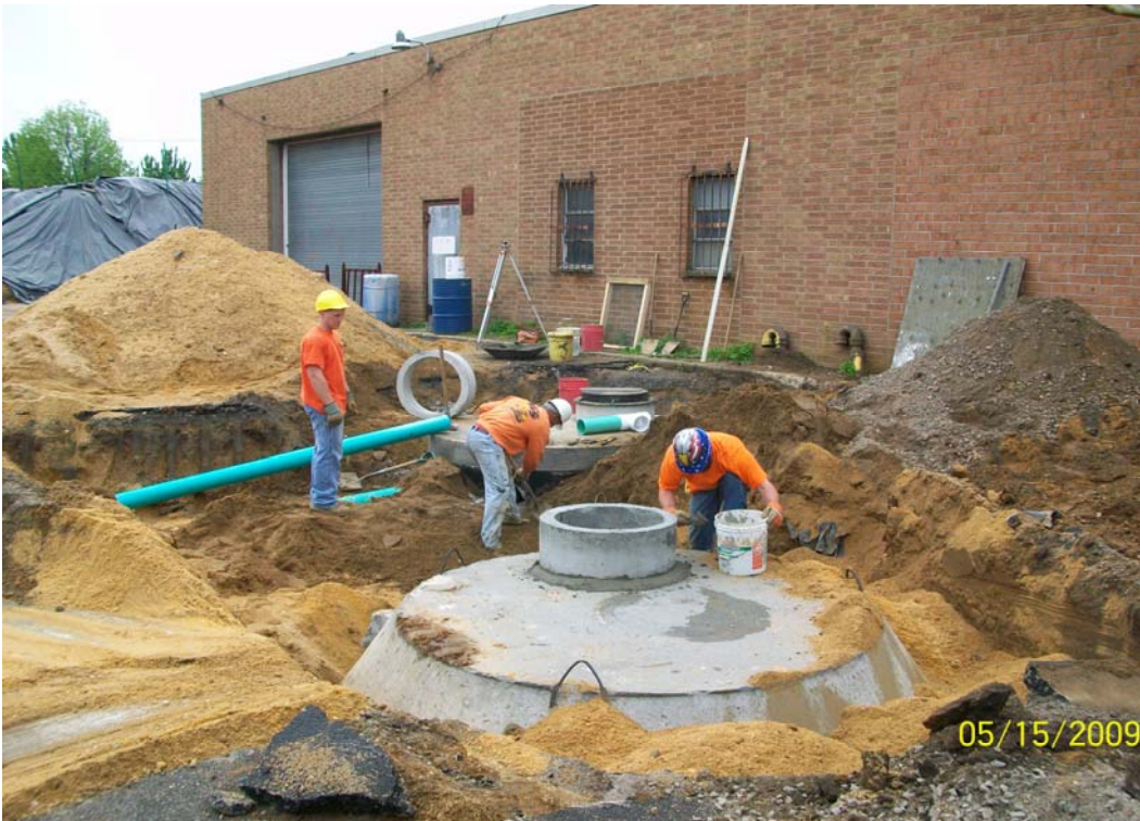
100_00611.jpg - Finished installing PCP-3B
