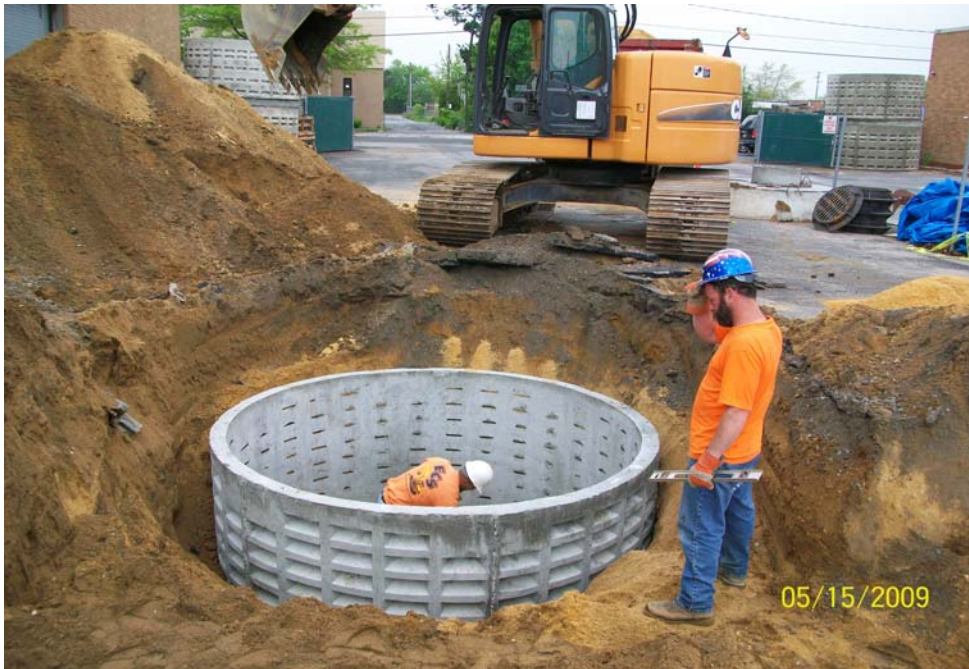
100_00610.jpg - Cork & Sons installing PCP-3B (51 Cabot St.)
