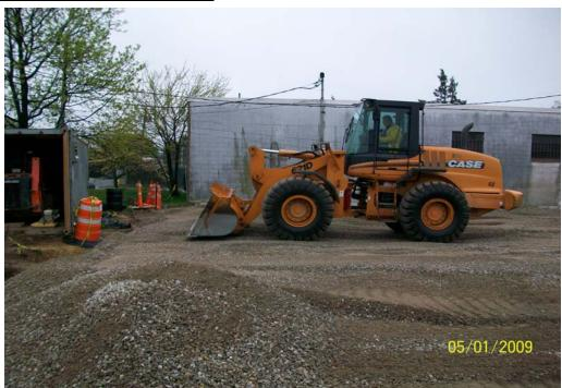
100\_00533.jpg - Spreading RCA to grade on excavation,
