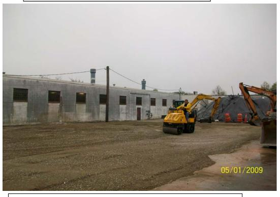
100\_00534.jpg - Compacting RCA to grade on excavation, looking SW
