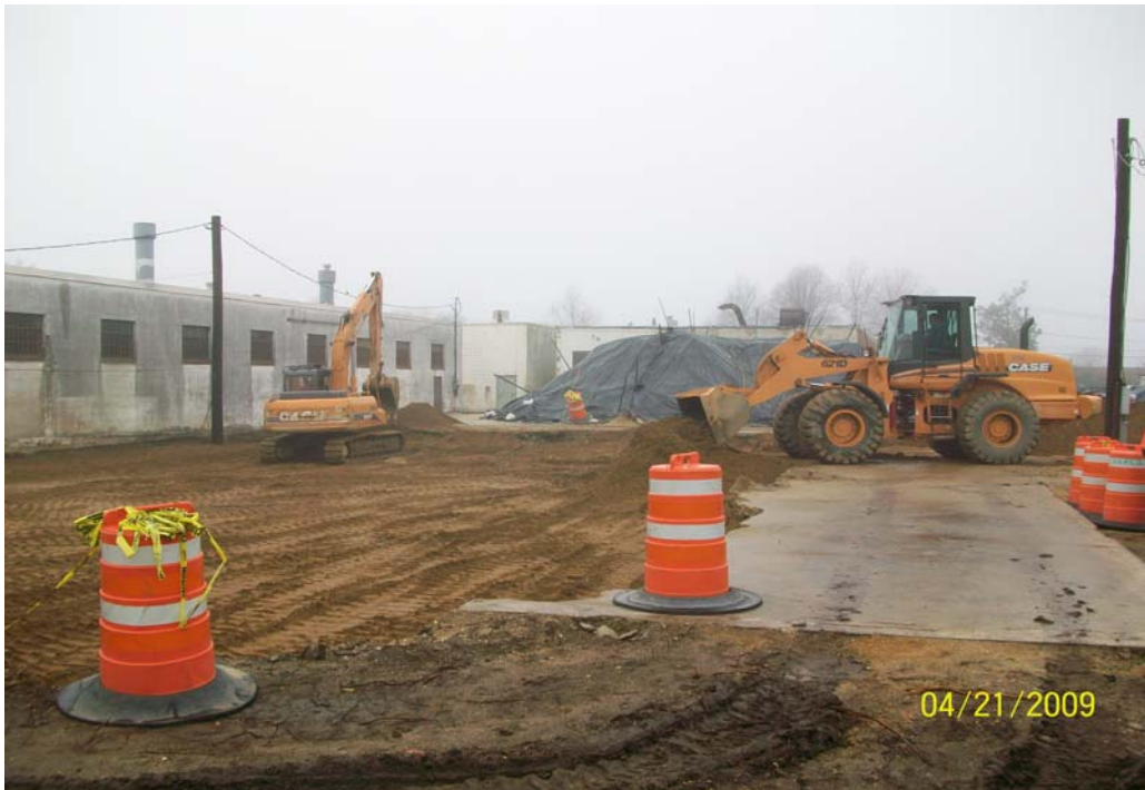
100_00442.jpg - Backfilling excavation, looking west.
