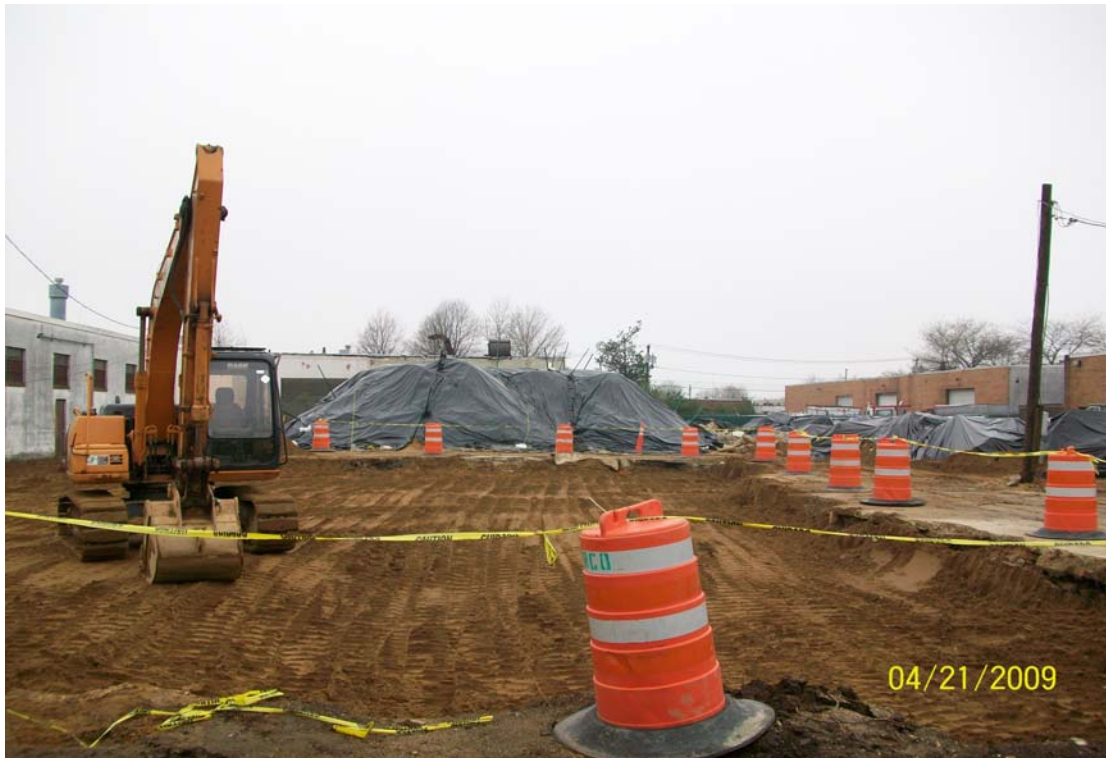
100_00445.jpg - Excavation at the end of the day, looking west
