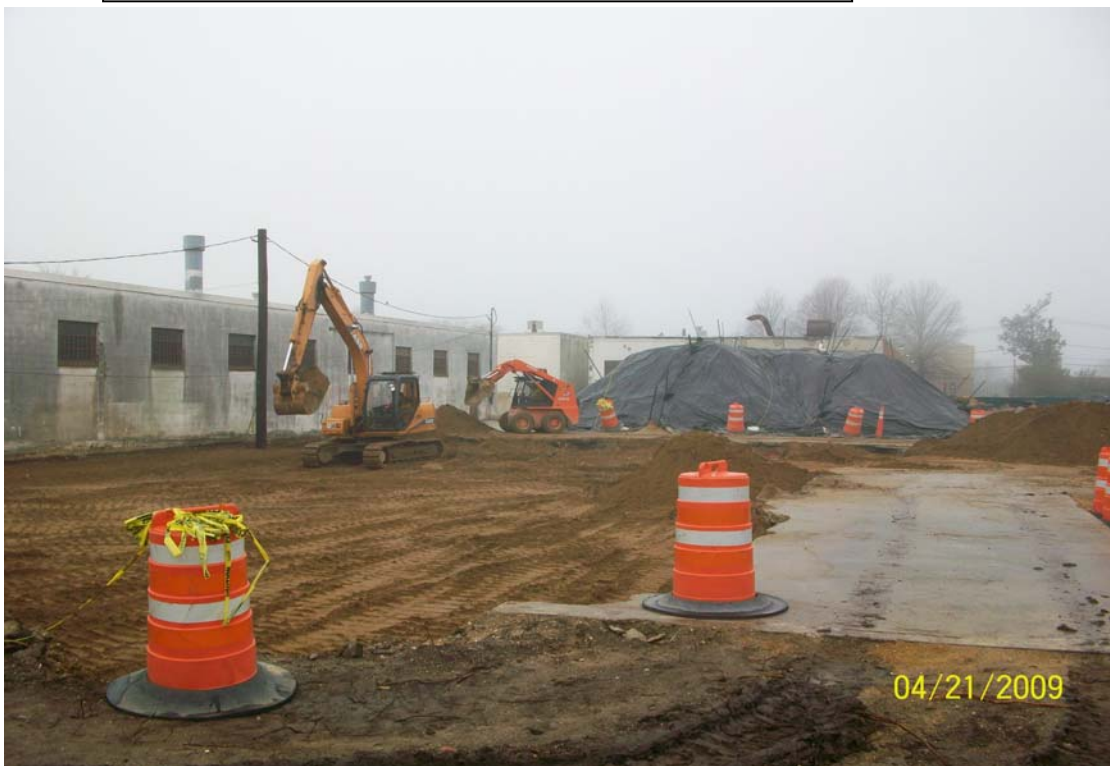
100_00443.jpg - Backfilling excavation, looking west
