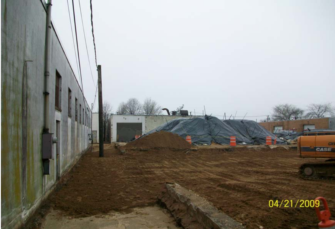
100_00444.jpg - Excavation at the end of the day, looking west
