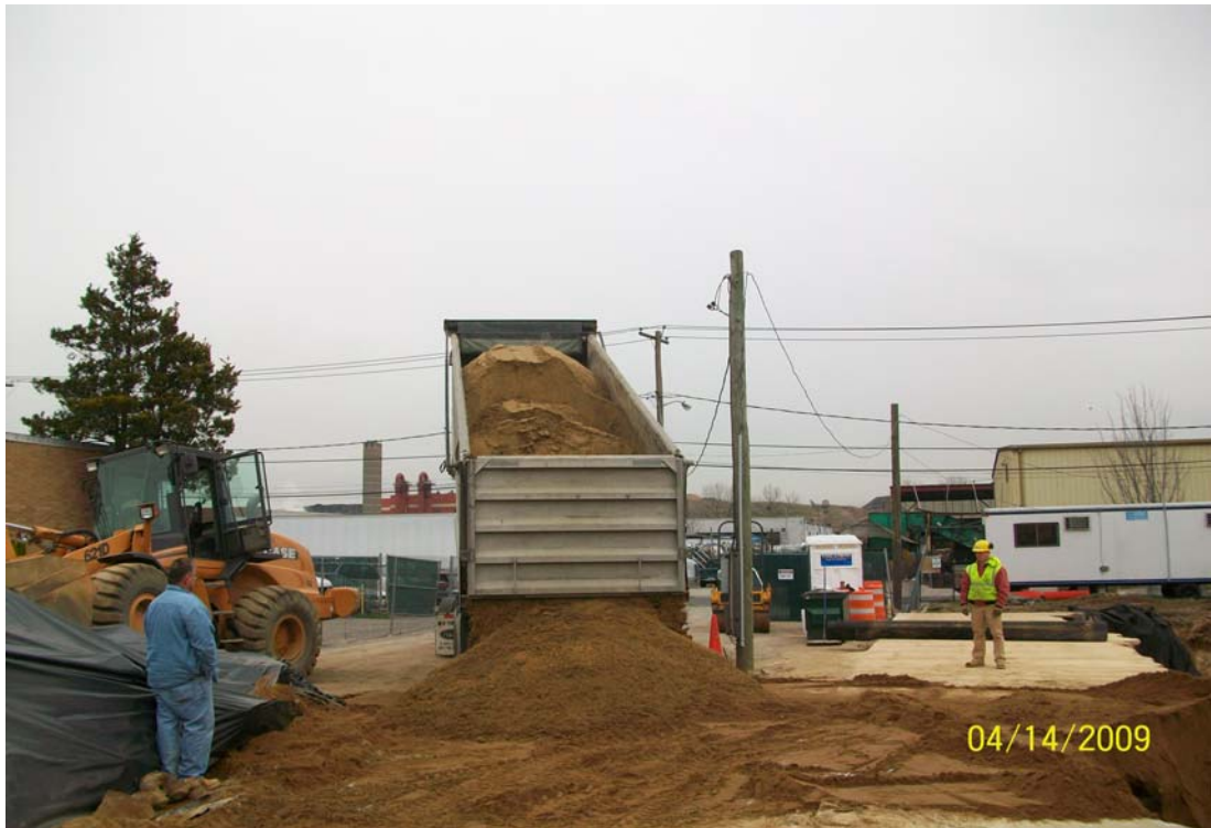
100_00358.jpg - Unloading backfill material, looking east
