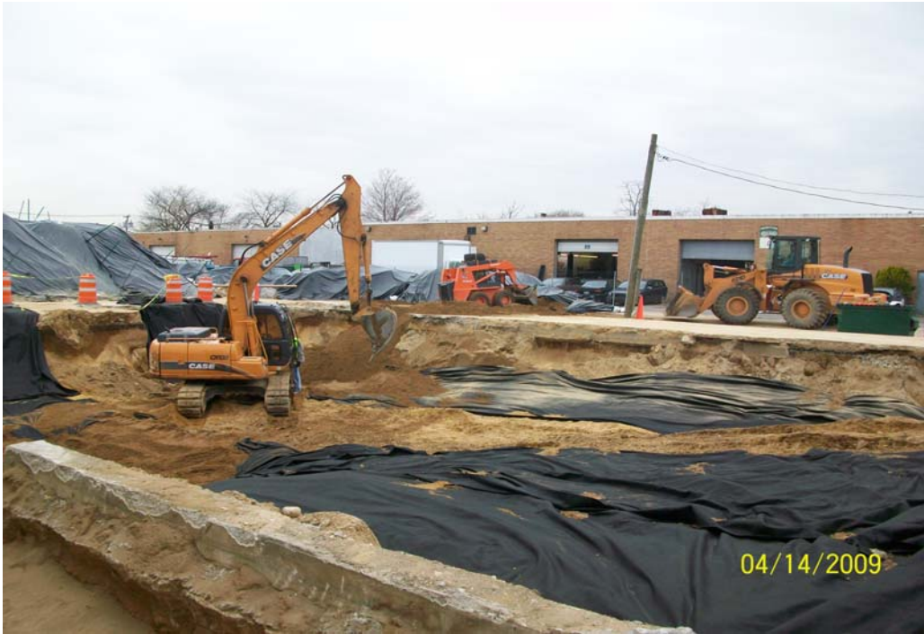
100_00356.jpg - Backfilling and compacting excavation, looking NW
