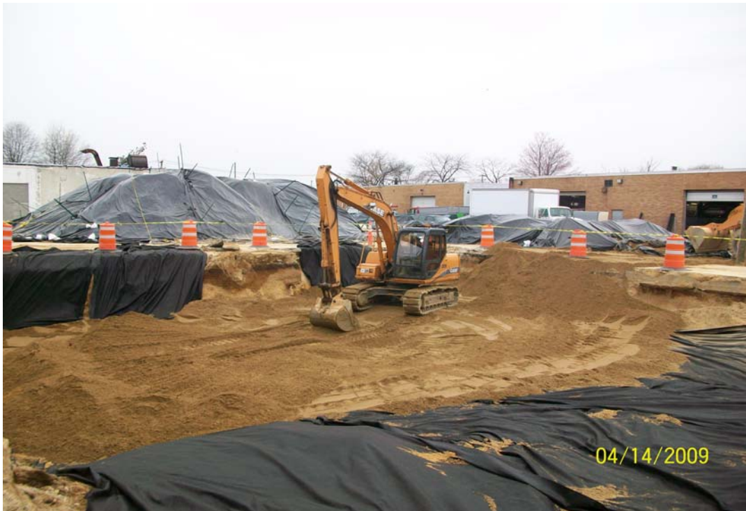
100_00360.jpg - Backfilling excavation at the end of the day, looking SW
