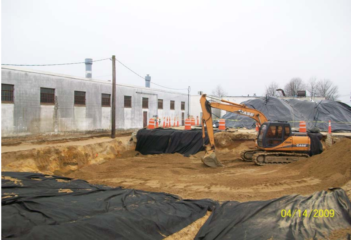
100_00359.jpg - Backfilling excavation at the end of the day, looking NW
