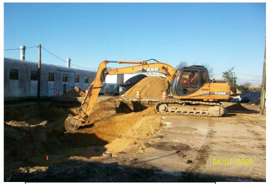
100\_00333.jpg - Excavator excavating ramp that was used to get to SEB-3/SES-5 area
