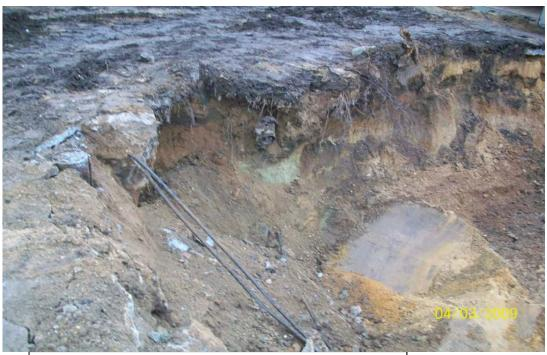
100\_00322.jpg - Green contaminated soil in NE corner of excavation
