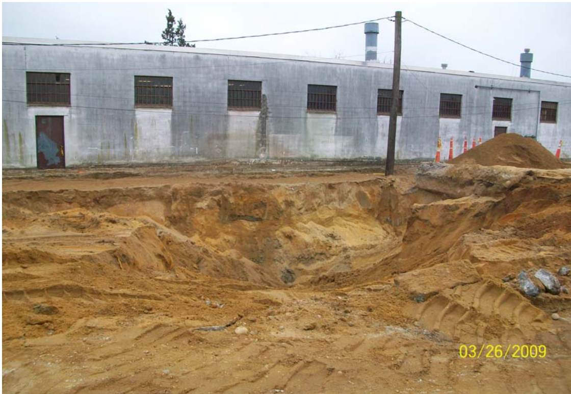
100_00224.jpg - Excavation at the end of the day, looking south.
