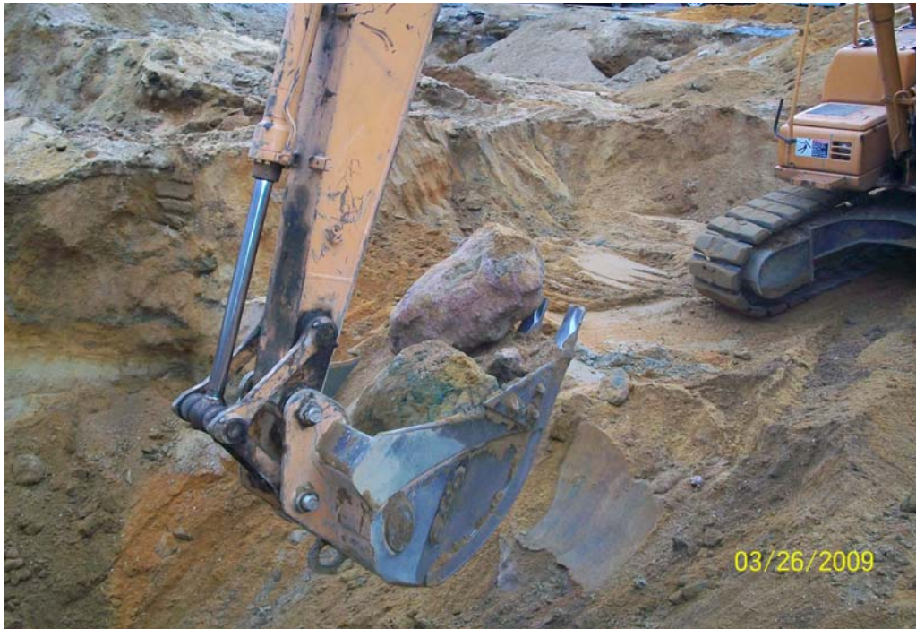
100_00215.jpg - Chunks of red and green contaminated material out of the area around sump-3
