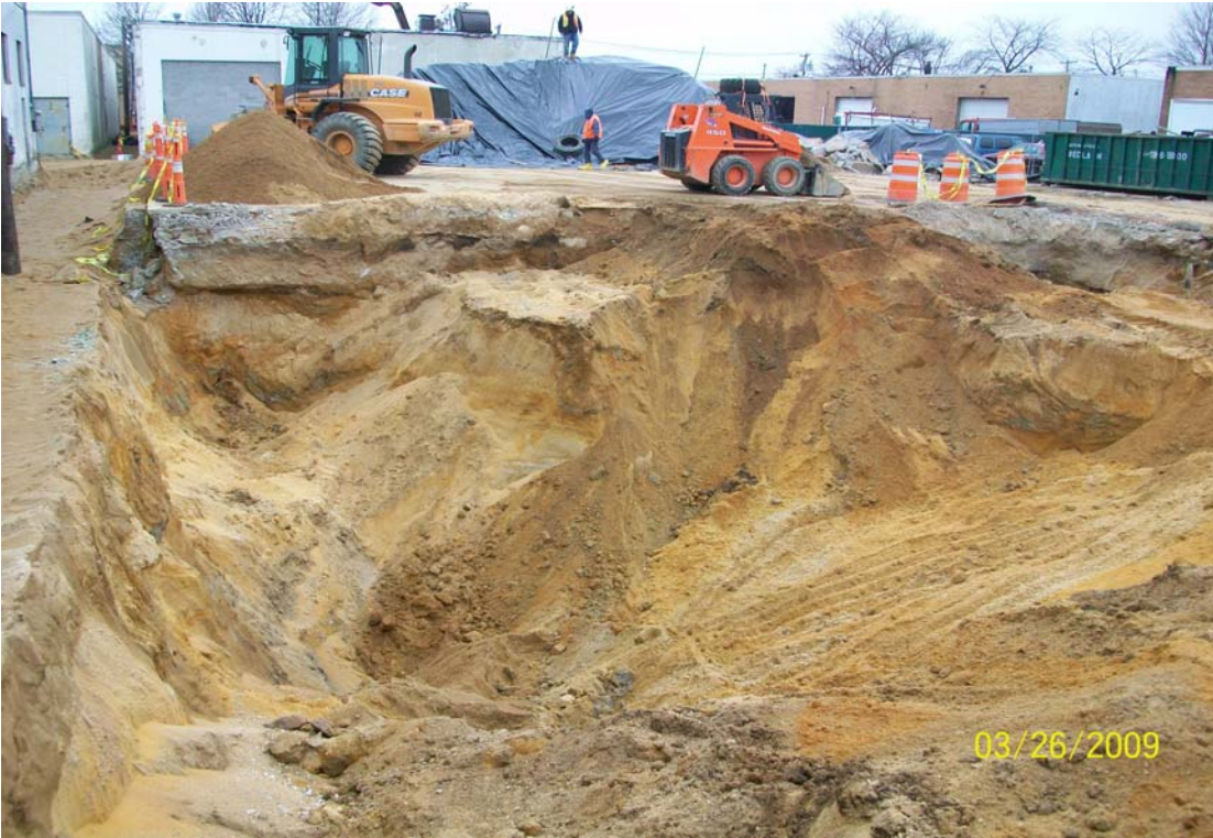
100_00225.jpg - Excavation at the end of the day, looking south.
