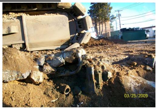
100\_00190.jpg - 3 PVC pipes found just below the slab. See drawing for location.
