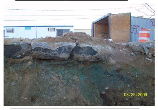
100\_00191.jpg - Green stained soil on east side of excavation
