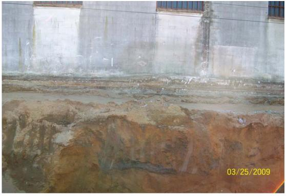
100\_00203.jpg - Green clay like material with red crust around, south side of excavation.
