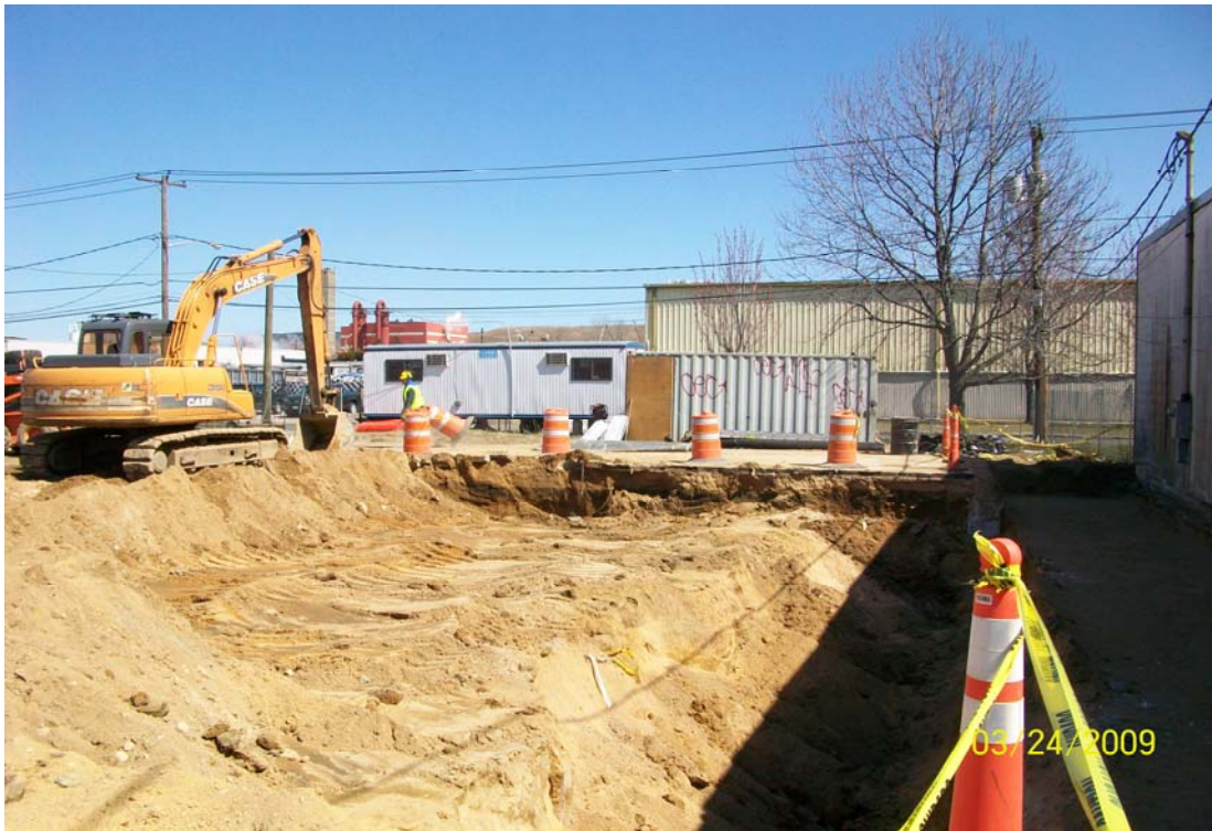
100_00182.jpg - End of day view of excavation.
