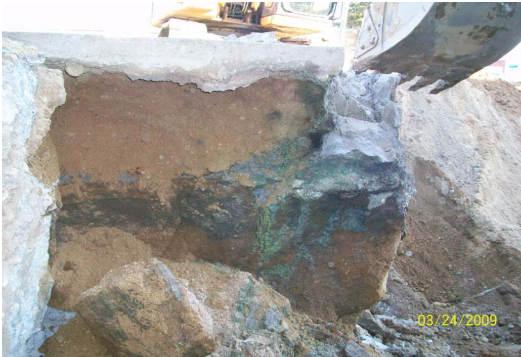
100_00168.jpg - Green stained concrete from the foundation wall.
