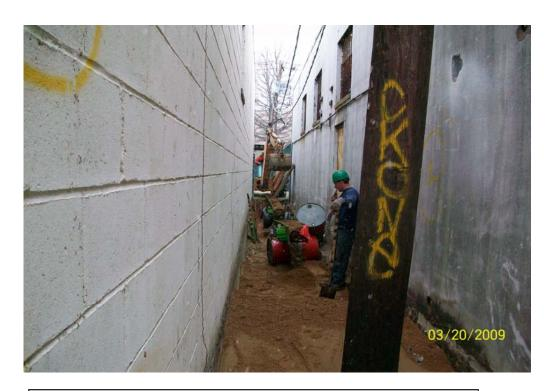
100\_00140.jpg - Backfilling and compacting west alleyway west of utility pole.
