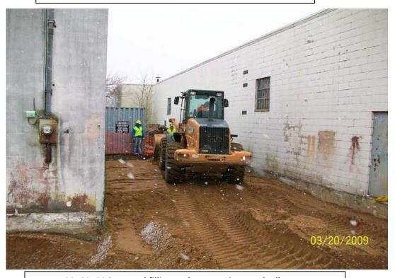
100\_00139.jpg - Backfilling and compacting south alleyway.
