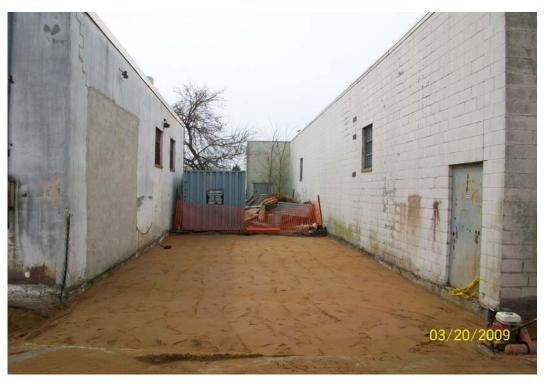
100 0041.jpg - Finished backfilling and compacting the south alleyway
