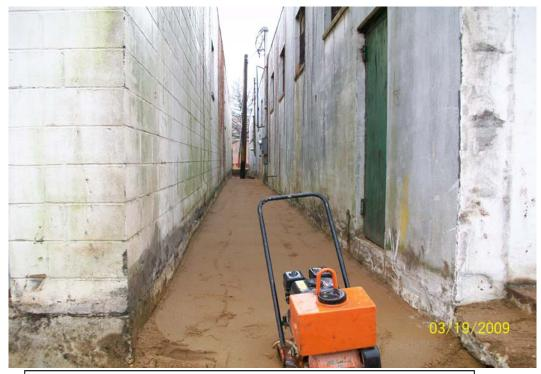
100\_00136.jpg - Finished backfilling and compacting the west alleyway from the utility pole east.
