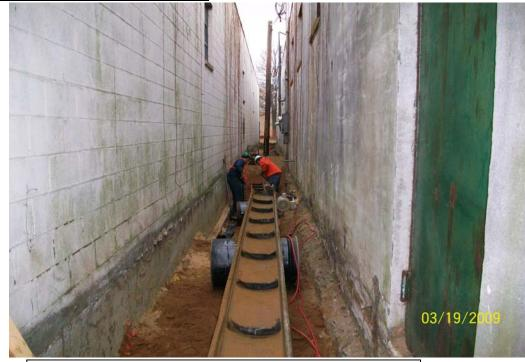
100\_00134.jpg - Backfilling and compacting west alleyway using conveyor to move the material.
