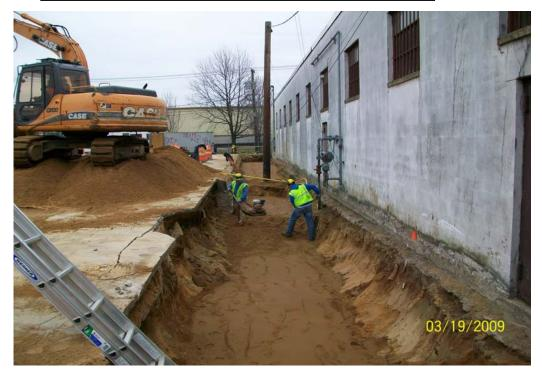
100\_00135.jpg - Backfilling and compacting the east alleyway.
