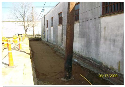
100\_00130.jpg - Backfilling and compaction completed for the day at the east alleyway, looking east.
