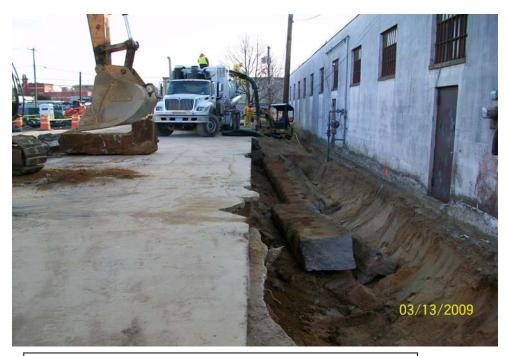
100\_00117.jpg - 50 Dale St. collapsed concrete wall being removed.
