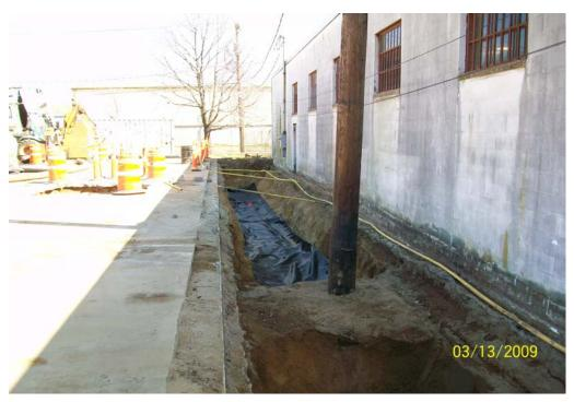
100\_122.jpg - Filter fabric on east alleyway excavation, looking east.
