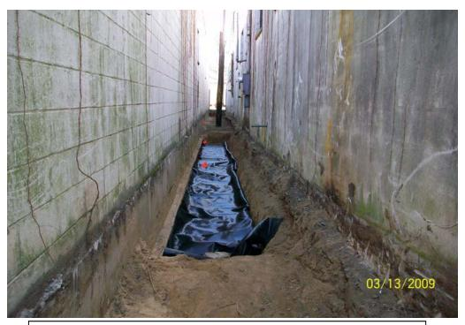
100\_0120.jpg - Filter fabric on west alleyway excavation. Flags are sample locations, looking west.
