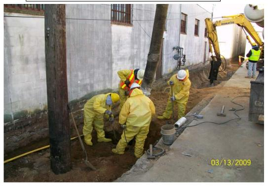
100\_0119.jpg - Excavating east alleyway with vac truck.
