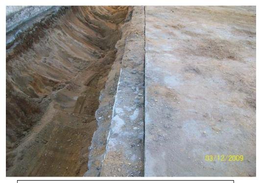
100\_0111.jpg - Crack separating 50 Dale St. slab from wall.
