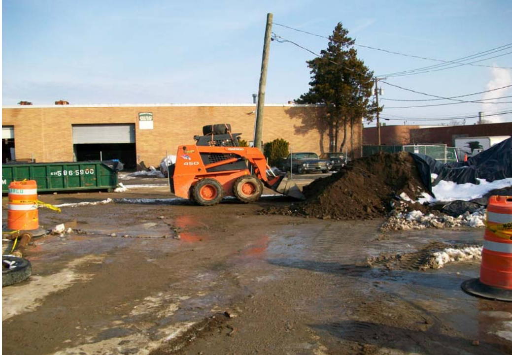
100_0018.jpg - Skid steer consolidating hazardous soil pile
