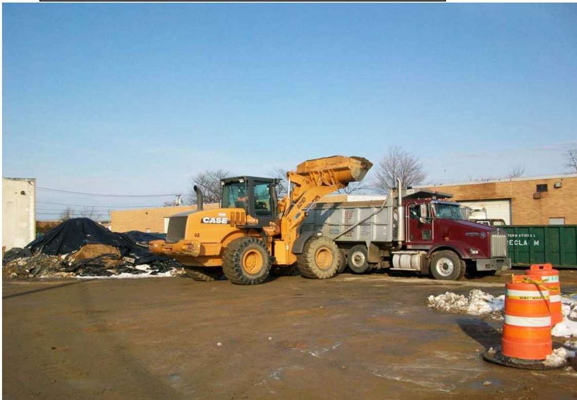
100_0016.jpg - Front end loader loading hazardous soil into a dump truck
