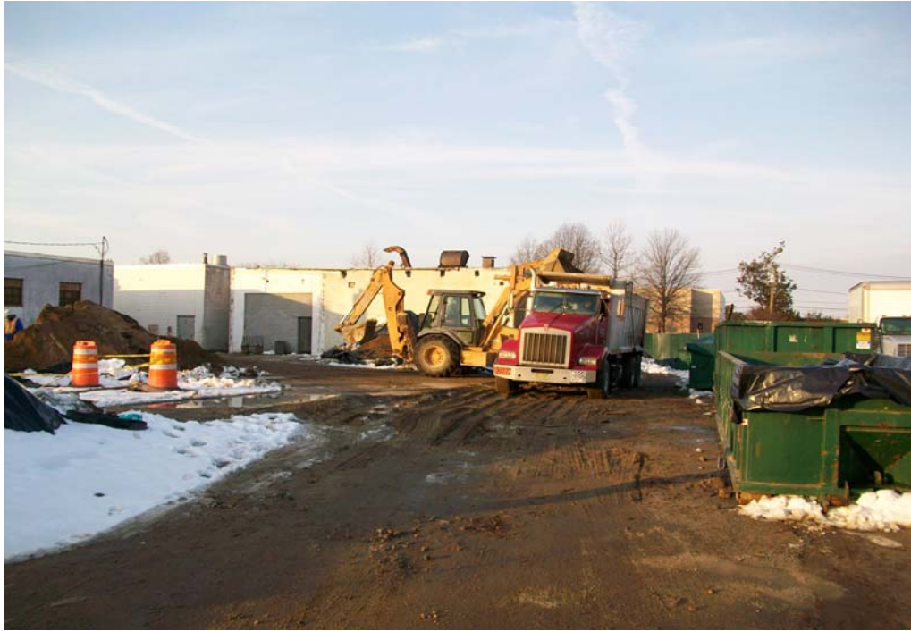
100_0015.jpg - Backhoe loading hazardous soil into a dump
