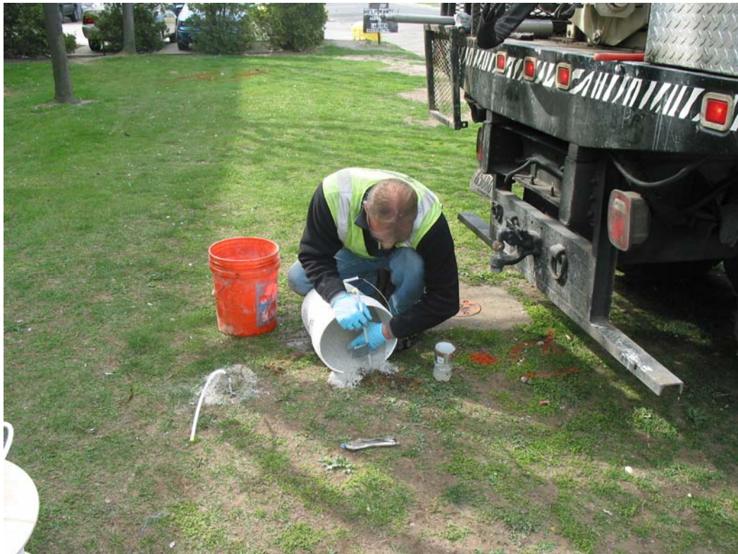
Installation of SV-12 across Dale Street from Spectrum
