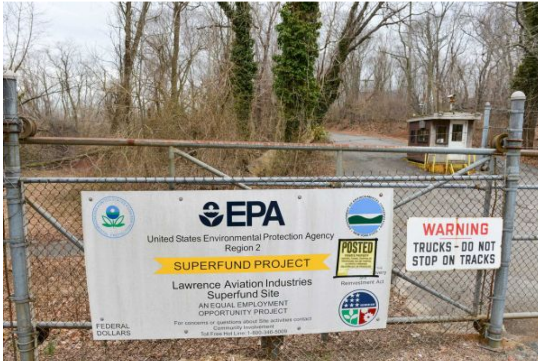
A view of the gated and fenced entry way into Lawrence Aviation Industries Inc. in Port Jefferson Station on April 2, 2014. (Credit: Daniel Brennan)
