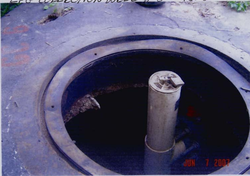
④ PG. 11 LFG COLLECTION WELL # 6 1 OF 2
