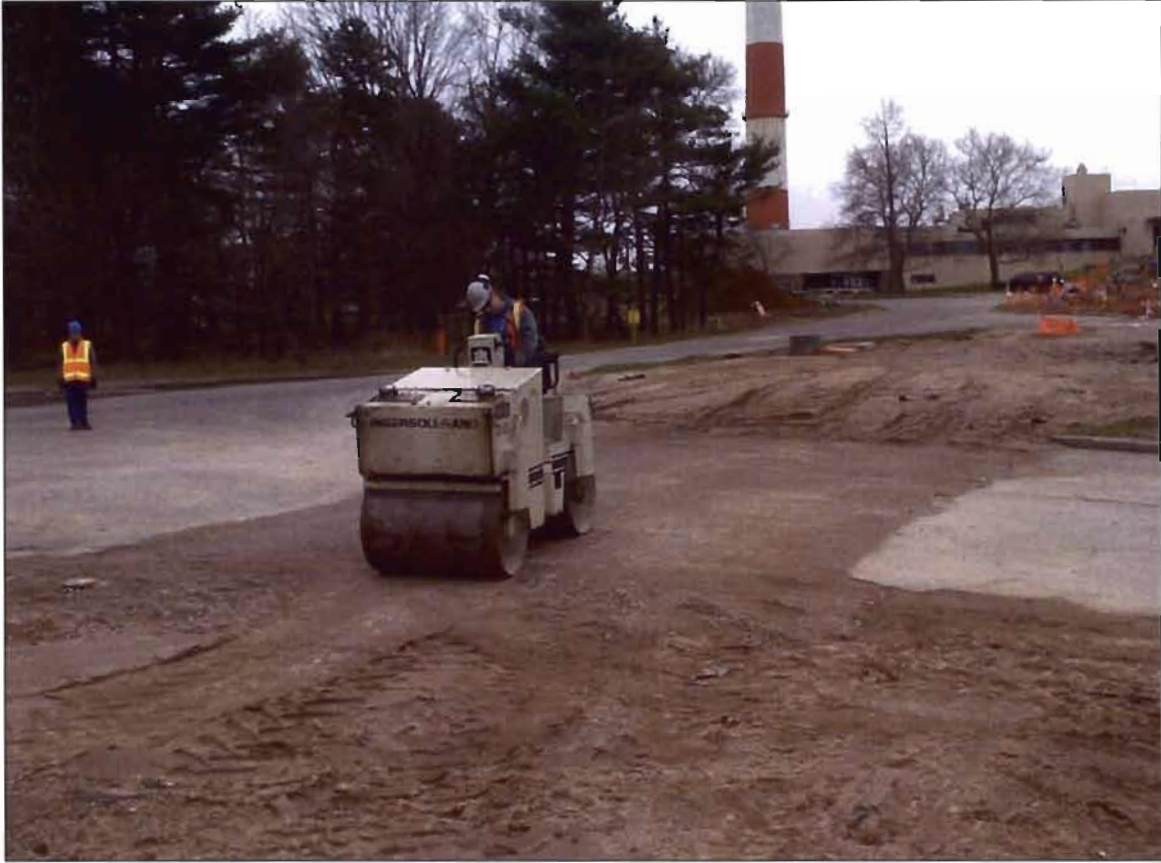
Photograph 6 – Site restoration (compaction) in Phase 4 of the Waste Transfer Lines
