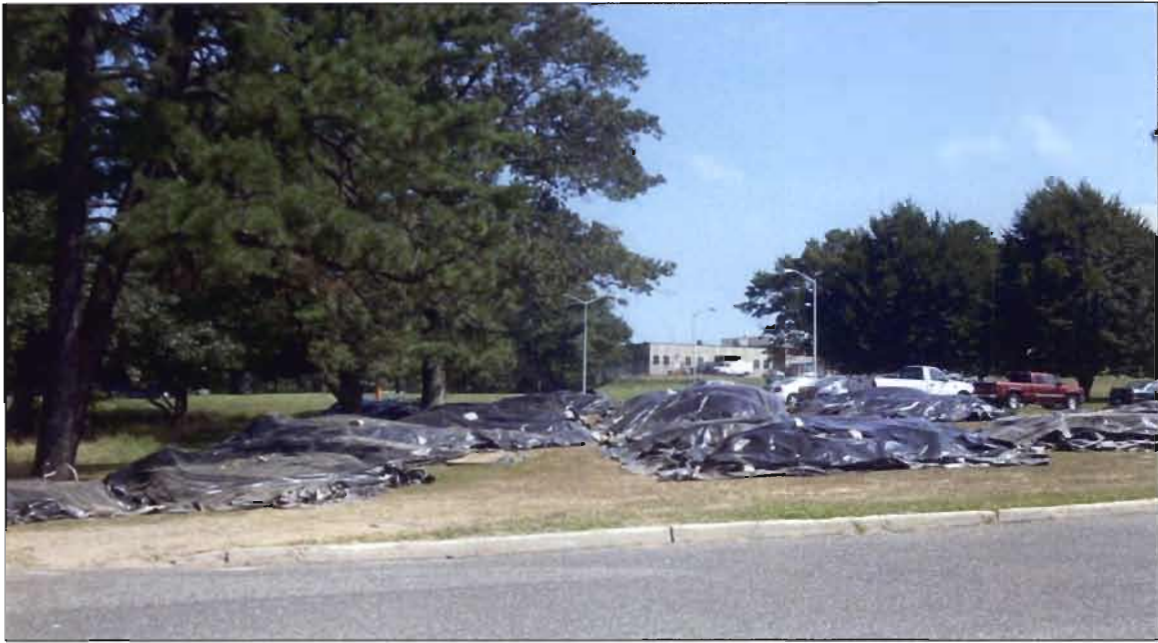
Photograph 2 – Overburden soil stockpiles at the Waste Transfer Lines site
