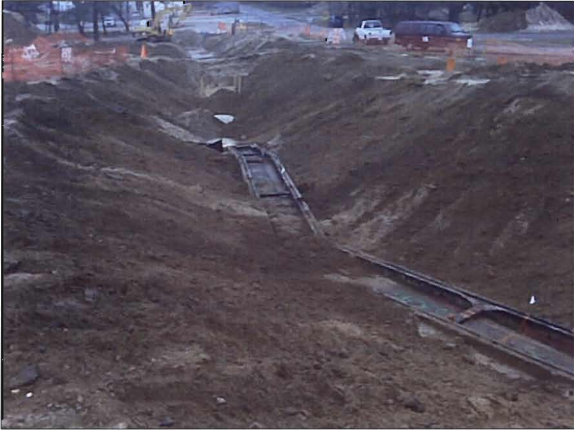
Photograph 4 – Segment of Phase 1 concrete culvert left in ground
