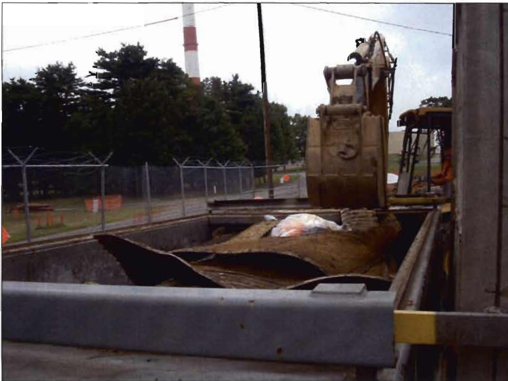
Photograph 5 – Packaging of Waste Transfer Lines debris.
