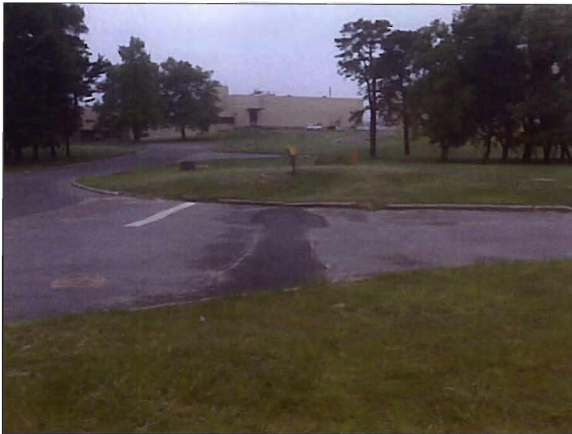
Photograph 1 – Pre-excitation conditions at the Waste Transfer Lines site (Phases 1–3)
