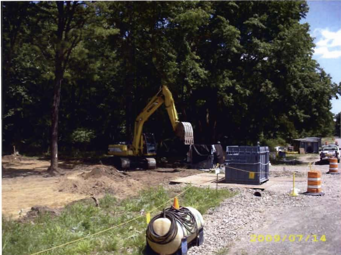
Photograph 2 – Soil removal at the former HWMF Perimeter Area.
