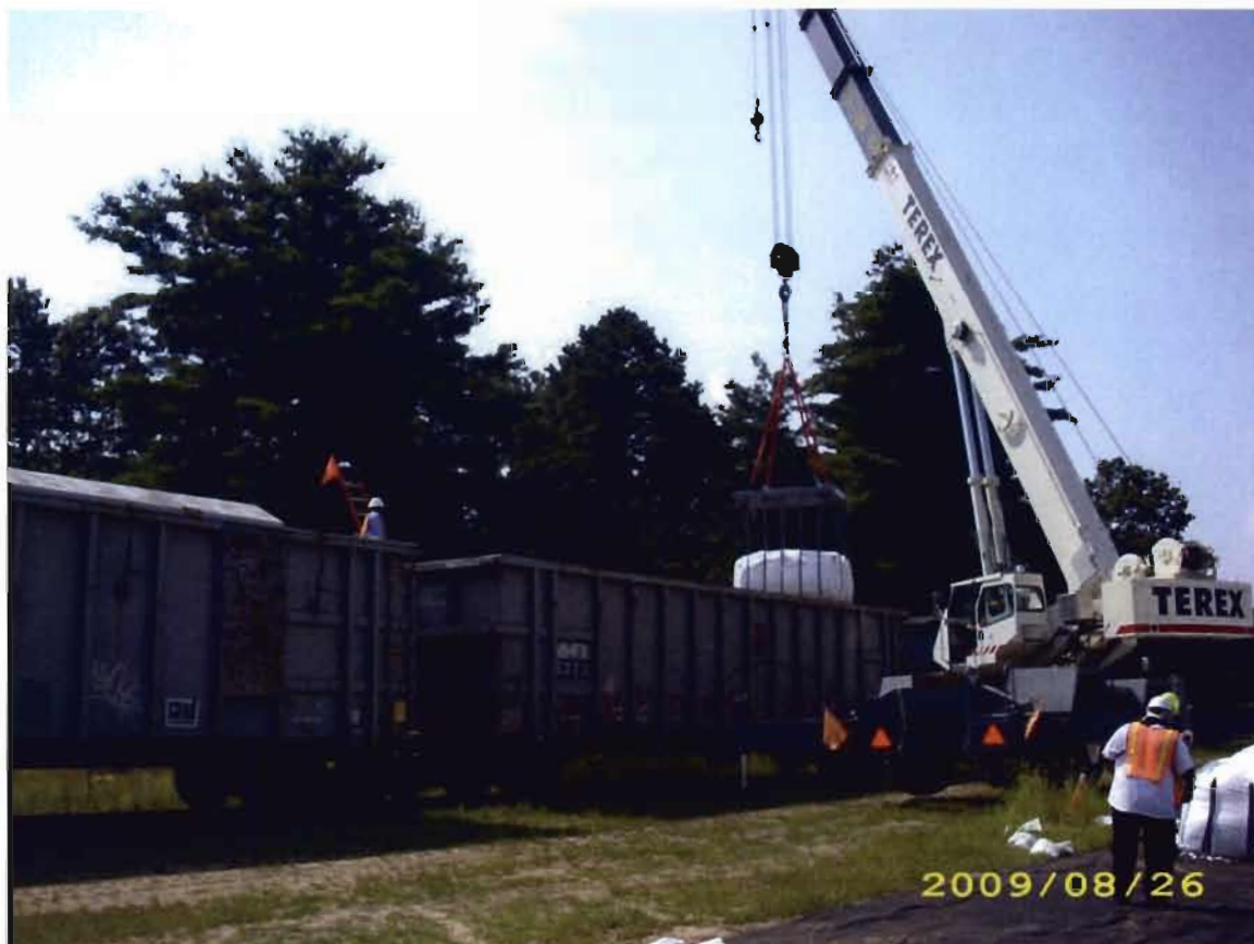
Photograph 3 – Loading Lift Liner containing contaminated soil into railcar at the WLA.
