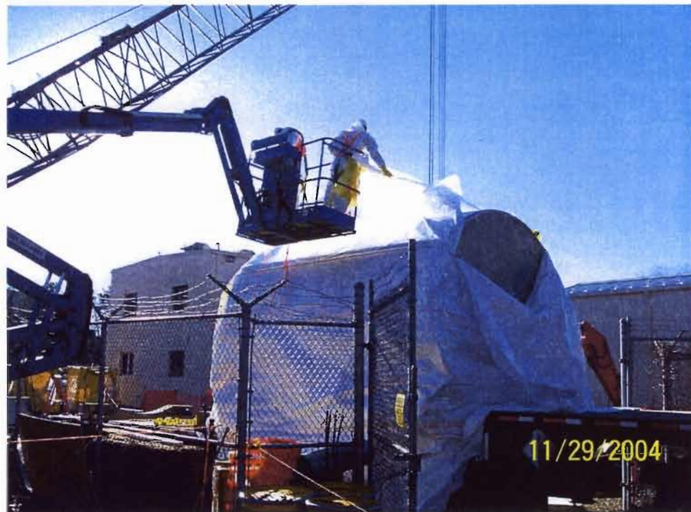
Photo 8: The USTs are loaded and crated for transport to Envirocare
