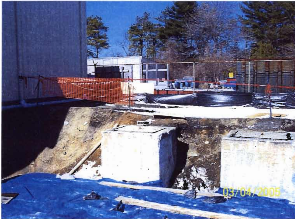
Photo 16: Valve pit covers were removed prior to cleanout
