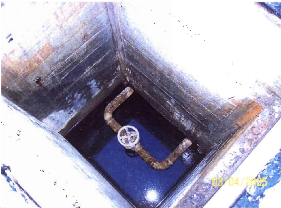
Photo 16: Valve pit covers were removed prior to cleanout
