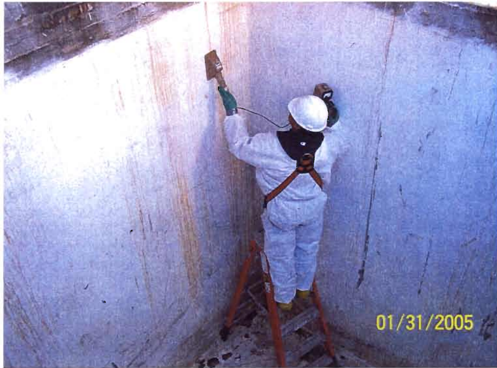
Photo 17: Vault walls are surveyed for radioactive contamination after clean-out
