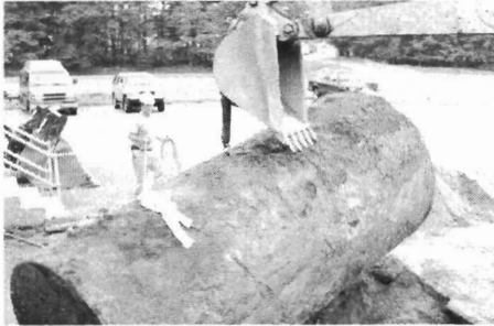
FIGURE 4. Removal of an empty underground storage tank.
