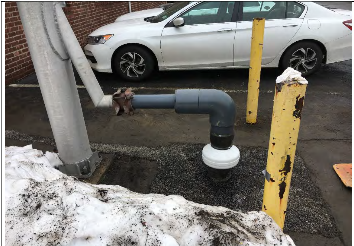
Photograph: 9 | Installed Fan, New Piping, Electrical Conduit & Temporary Asphalt Patch
