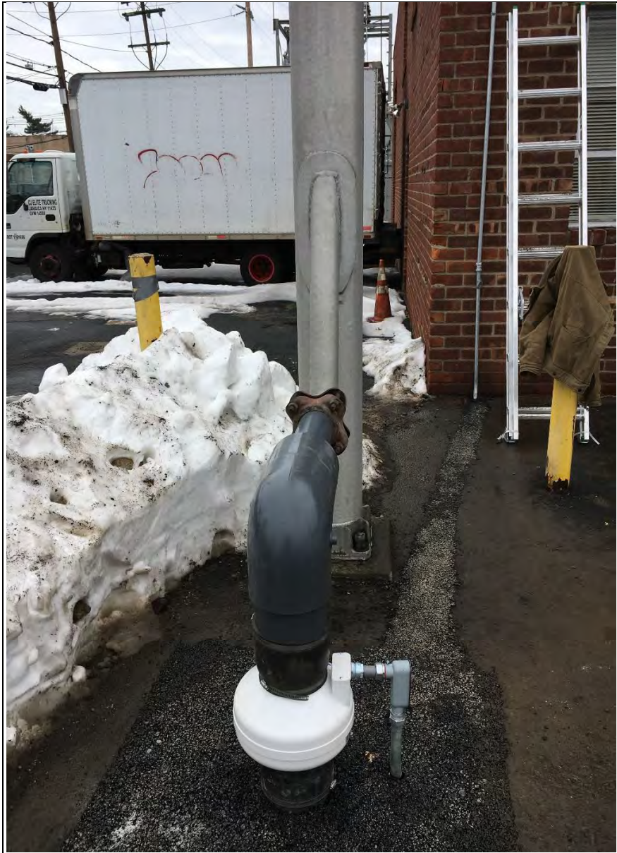
Photograph: 11 Installed Fan, New Piping, Electrical Conduit & Temporary Asphalt Patch
