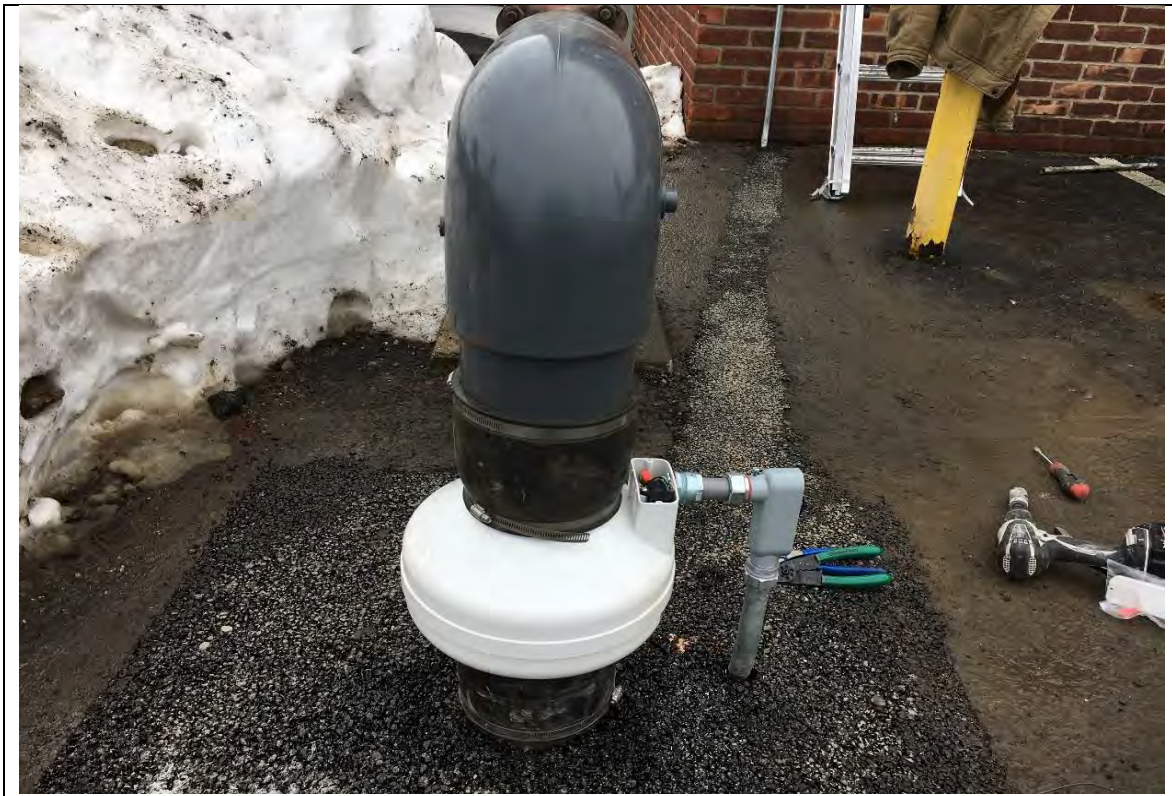
Photograph: 8 | Installed Fan, New Piping, Electrical Conduit & Temporary Asphalt Patch
