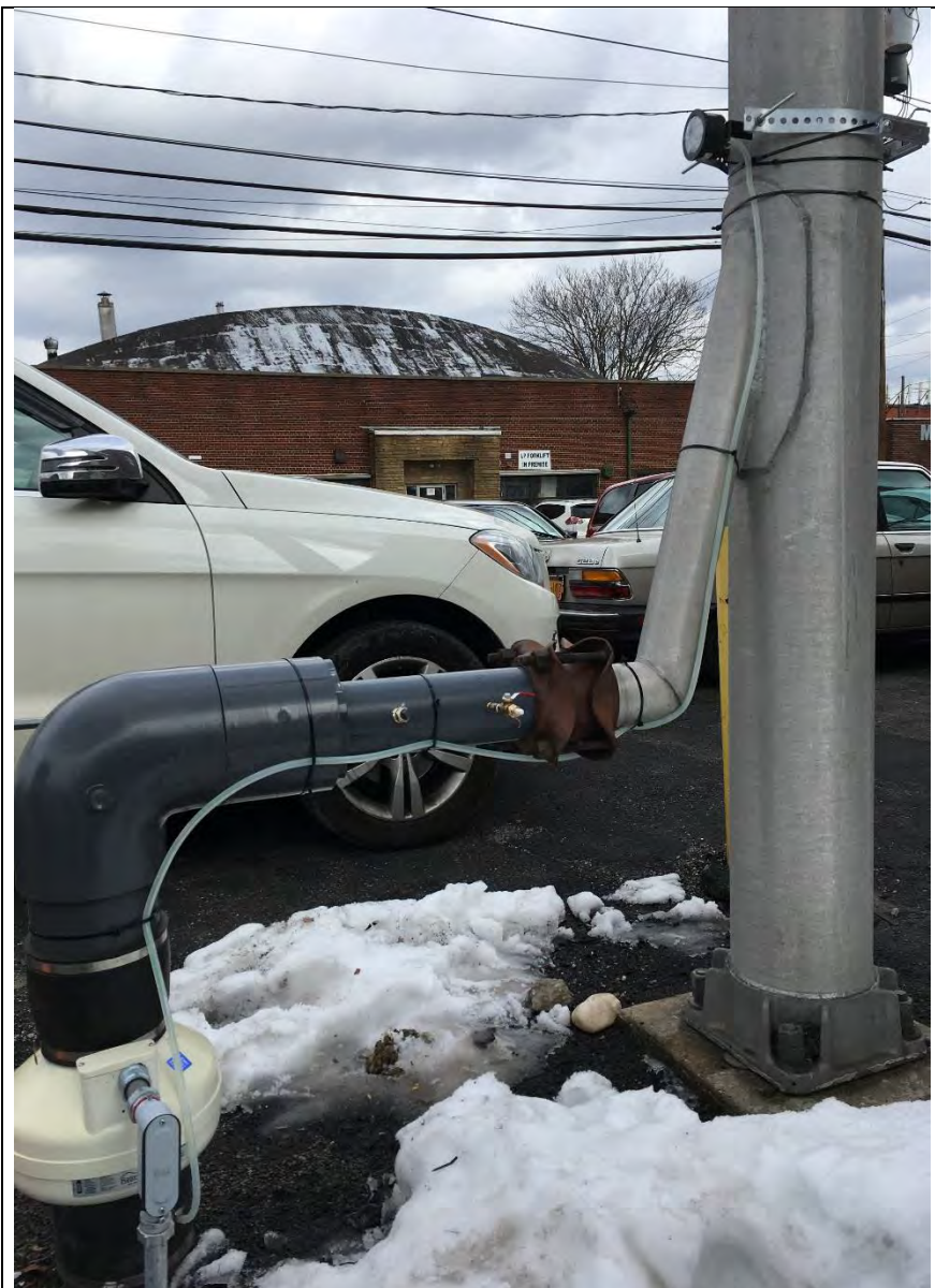
Photograph: 15 Installed Sample Port, Flow Measurement Port and Vacuum Gauge
