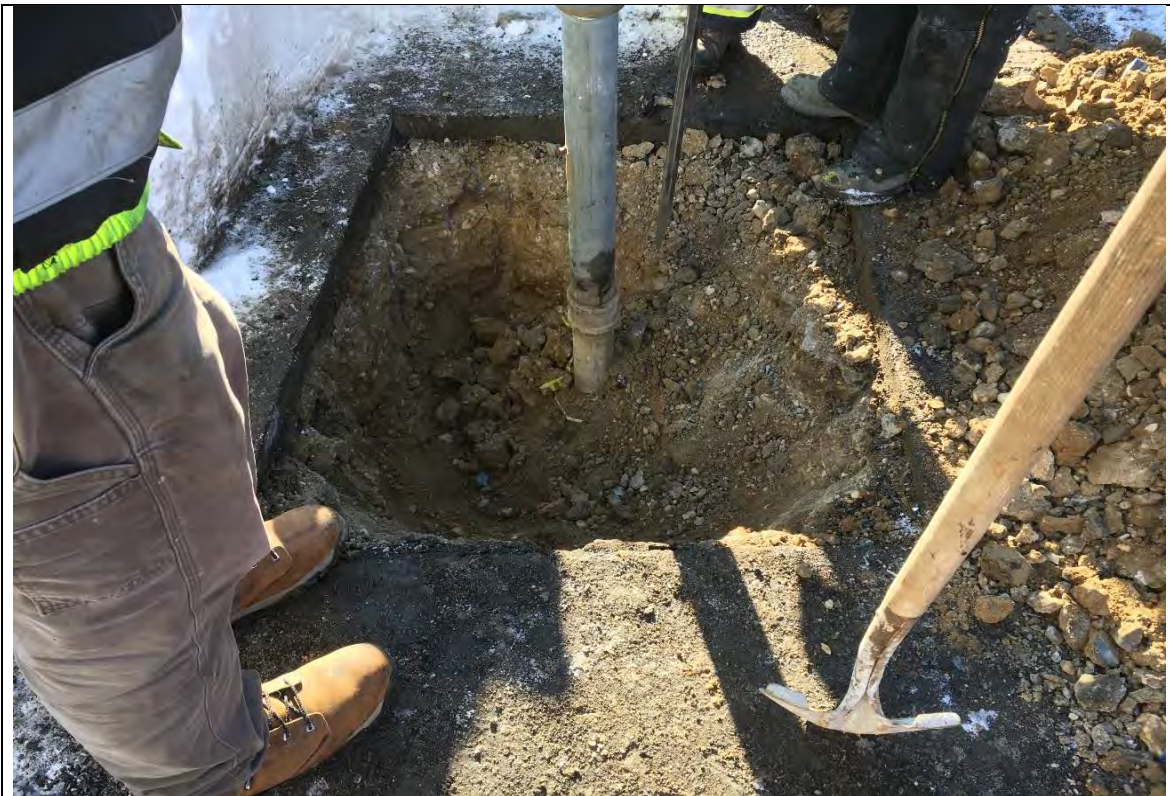
Photograph: 4 Excavation To Pipe Union In Order To Modify Piping For Fan Installation
