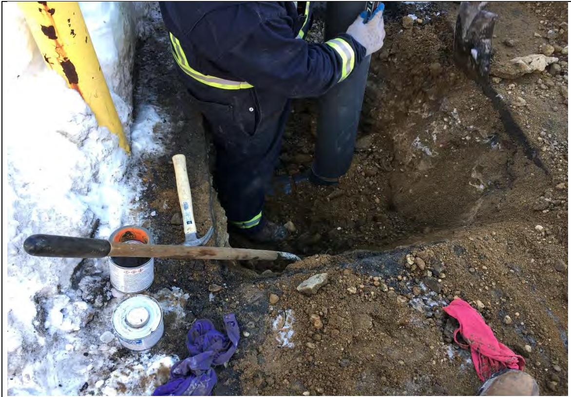
Photograph: 5 Confirming Plumb of Piping Modification For Fan Installation
