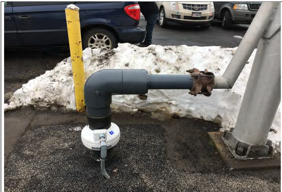
Photograph: 10 | Installed Fan, New Piping, Electrical Conduit & Temporary Asphalt Patch
