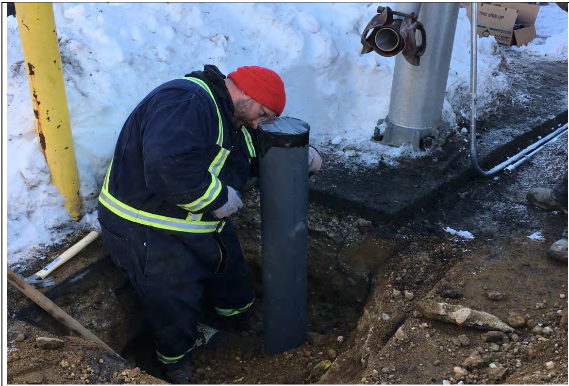
Photograph: 6 Confirming Plumb of Piping Modification For Fan Installation
