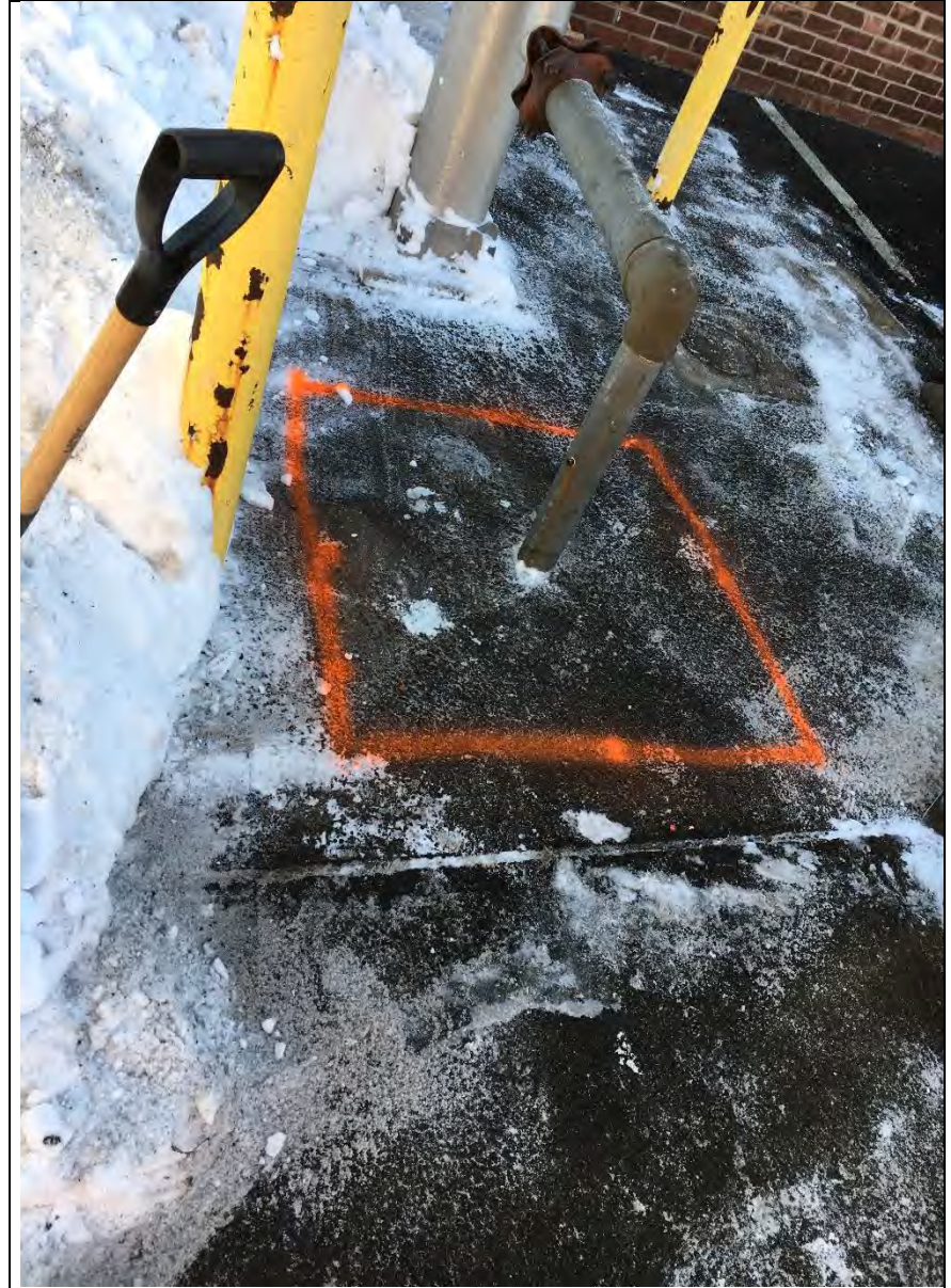
Photograph: 2 Excavation Area To Modify Piping For Fan Installation
