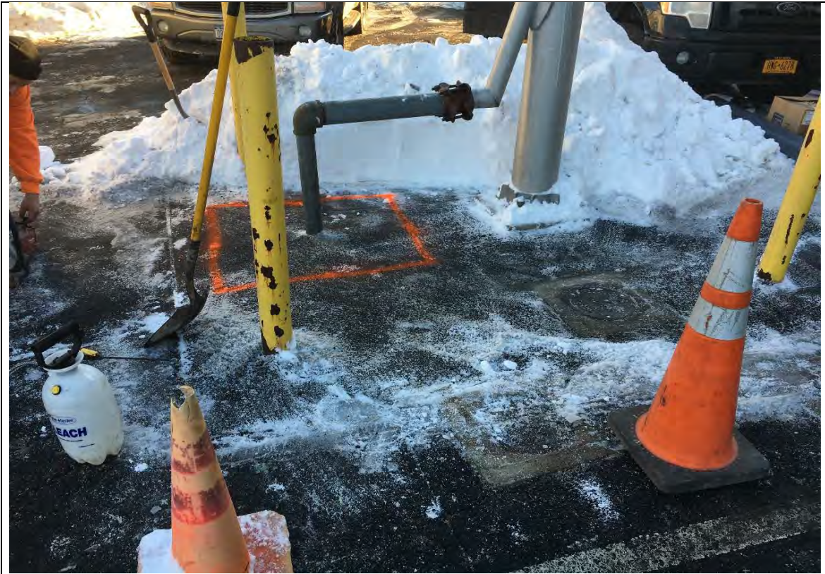
Photograph: 3 Work Area To Modify Piping & Install Fan
