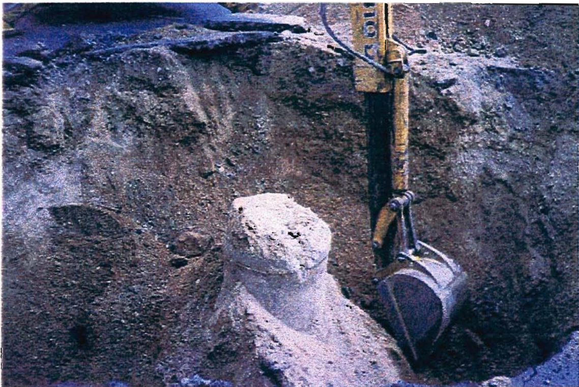
Excavation Of Top Cone
