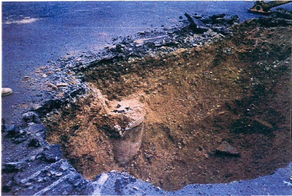
Dry Well Manway
