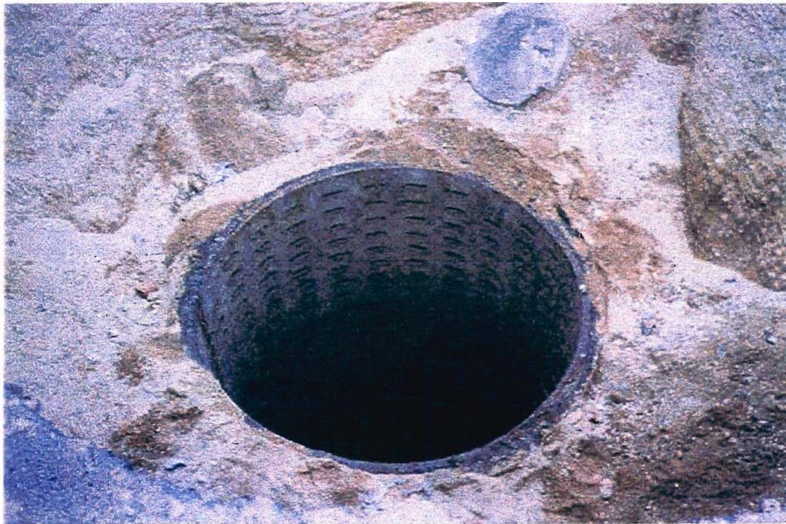
Dry Well With Top Cone Removed
