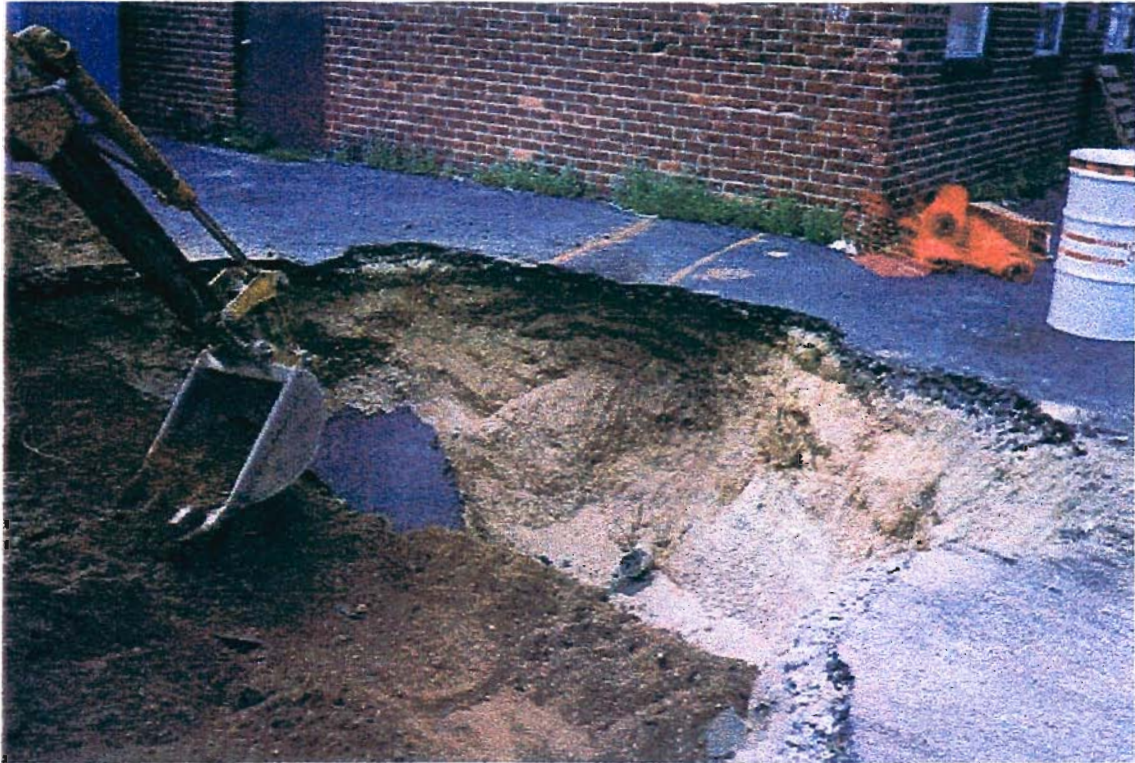
Sealed Drain Pipe And Backfill Of Excavation
