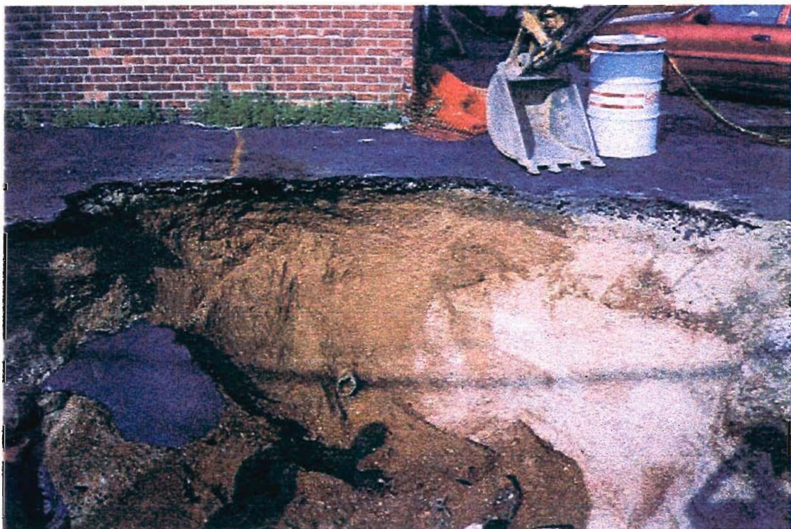
Drain Pipe Position Relative To NE Building Corner
