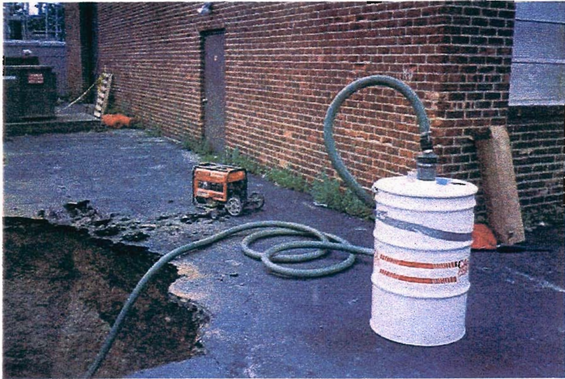
Treatment Of Dry Well Vapors Prior To Removal Of Top Cone
