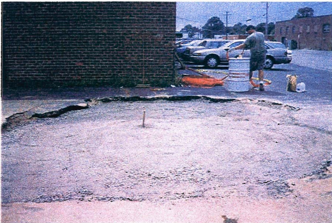
Gravel Base And Stake Showing Location Of Dry Well Center
