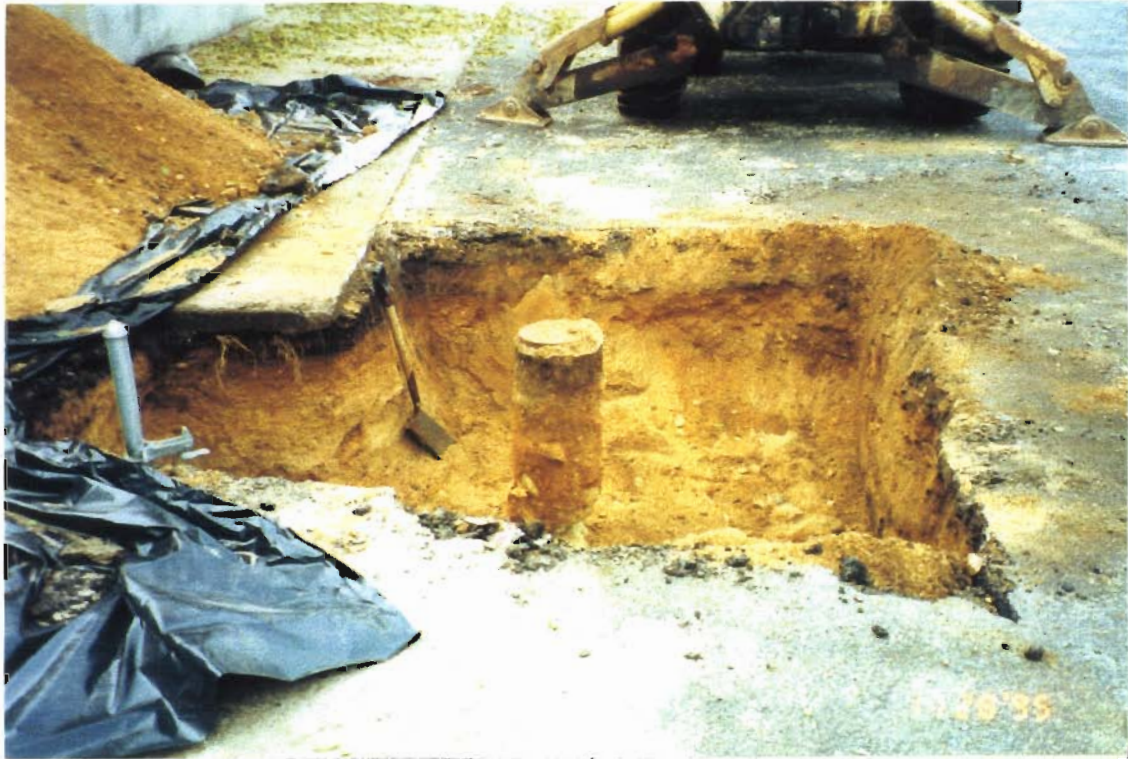
PHOTOGRAPH # 9 : Looking West at Completed Excavation.
