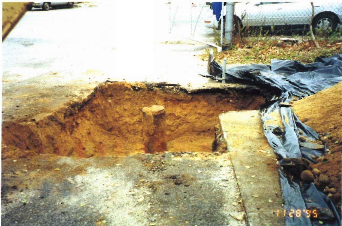
PHOTOGRAPH # 8 : Looking East at Completed Excavation.
