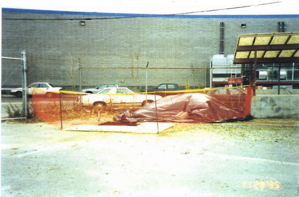
PHOTOGRAPH #12: Excavation Secured with Fencing, Plywood, and Yellow Caution Tape.
