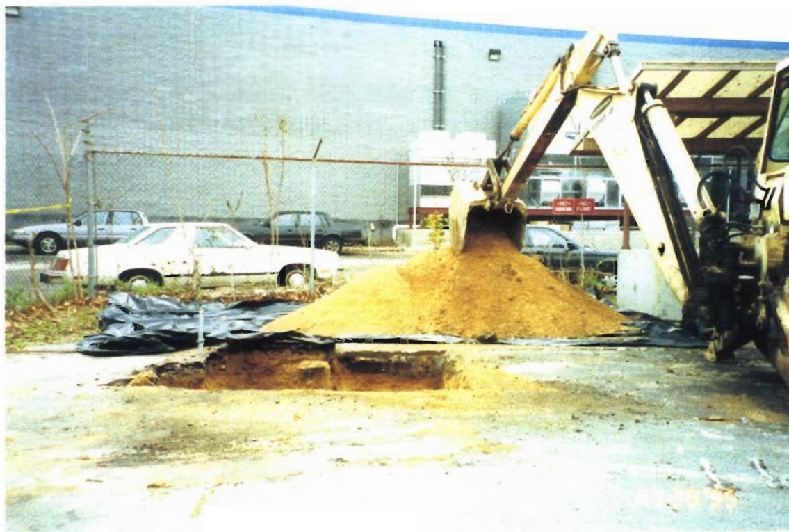
PHOTOGRAPH # 5 Excavation Completed. Looking South towards Photocircuit Building.
