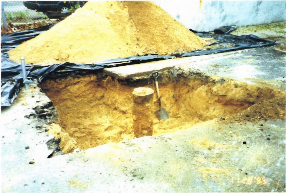
PHOTOGRAPH # 7 : Looking South at Completed Excavation.
