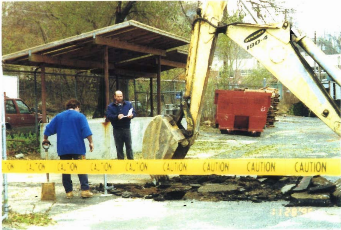
PHOTOGRAPH # 1 : Removal of Asphalt Top. Looking West.
