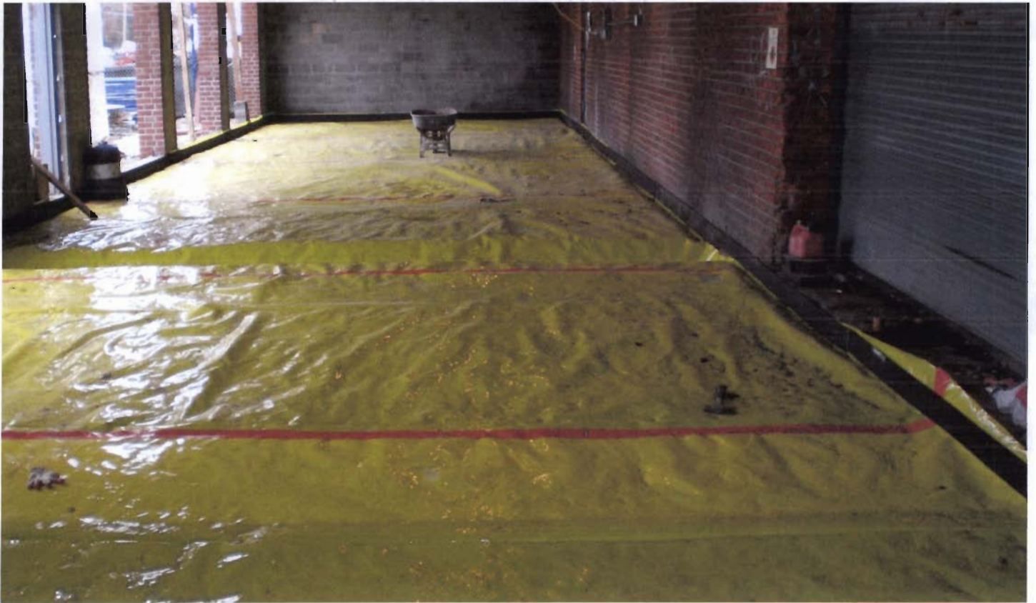
Photograph of vapor barrier
