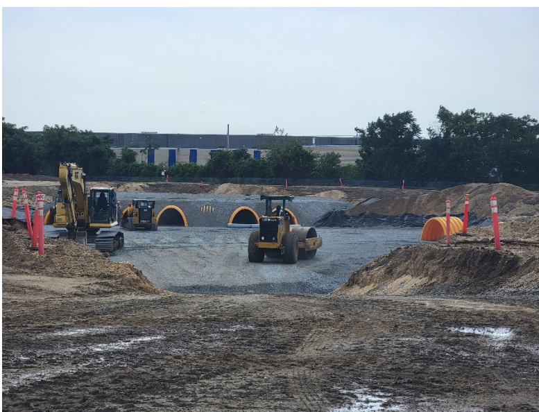
Photo 2: Looking south, Pratt continues the installation of drainage basin structures.
