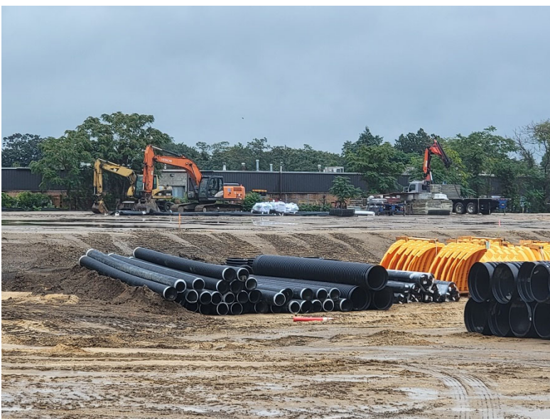
Photo 4: Ruttura begins mobilizing to site.
