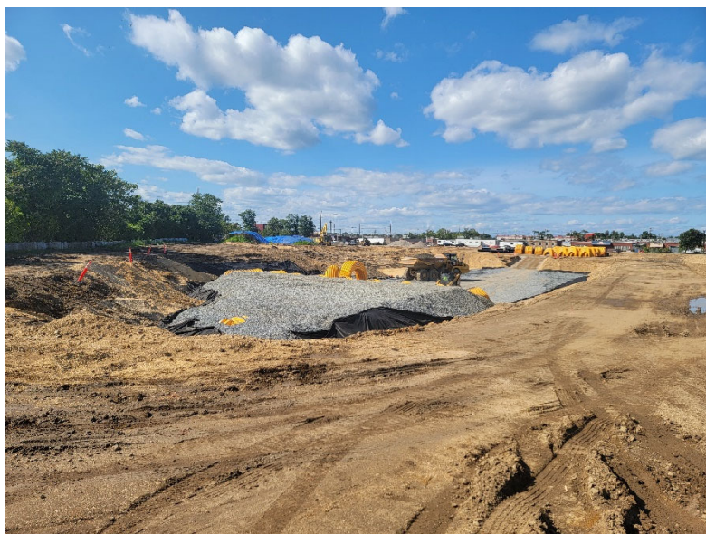
Photo 2: Looking northwest, Pratt continues the installation of drainage basin structures.
