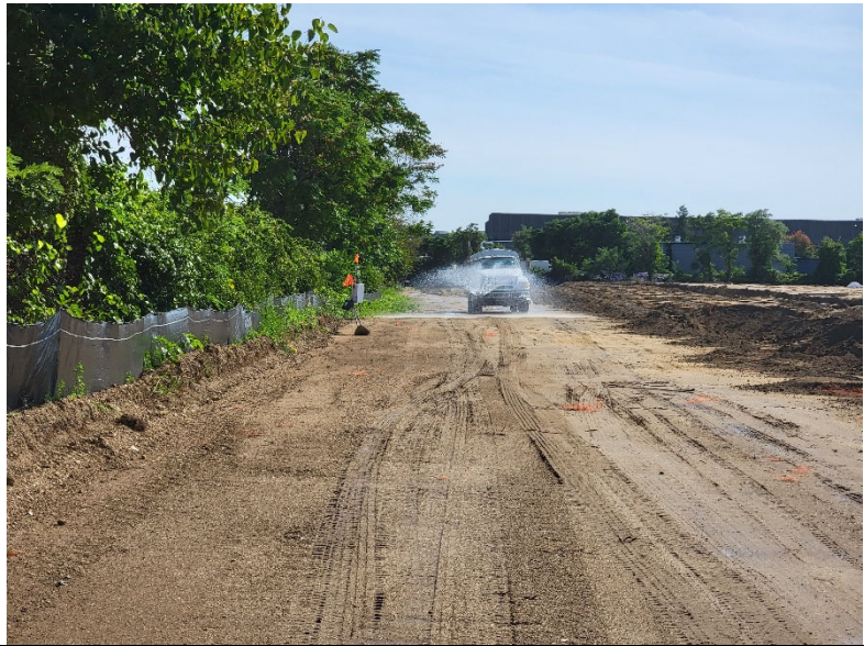
Photo 1: Looking south, view of CAMP Station 3 and active water truck being used for dust suppression throughout workday.
