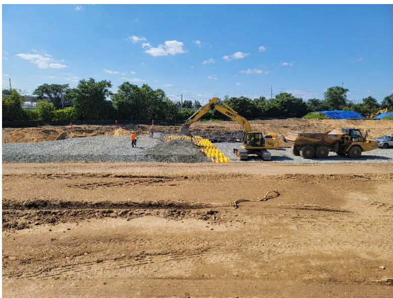
Photo 2: Looking west, Pratt continues the installation of drainage basin structures.
