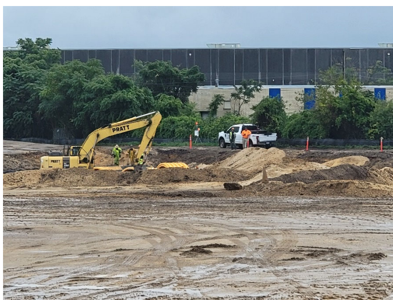
Photo 2: Looking southwest, Pratt begins the installation of drainage basin structures.
