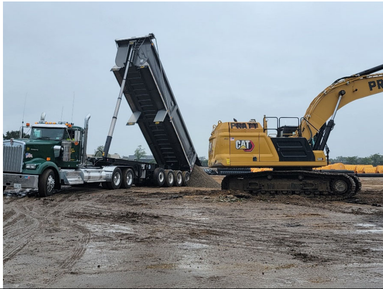
Photo 1: Looking east, Pratt receives RCA from South Shore.
