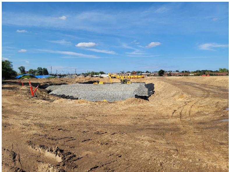
Photo 2: Looking north, Pratt continues the installation of drainage basin structures.
