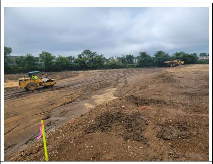
**Photo 3:** Looking southwest, Pratt continues regrading and compaction work on southern end of site.
