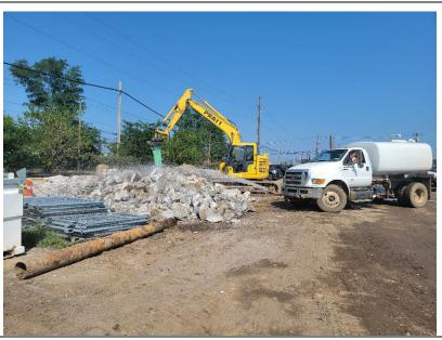
**Photo 1:** Looking northwest, Pratt begins breaking up concrete stockpiles for offsite disposal. The water truck is used for dust mitigation.
