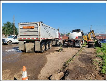
**Photo 1:** Looking north, Pratt uses power washer and truck pads to clean trucks post loading for dust mitigation and sediment track out control.
