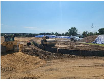
**Photo 4:** Looking south, Pratt continues regrading/drum rolling for soil compaction. Water truck in distance mitigating dust.
